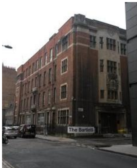
Figure 3 – Photograph of Former Royal Ear Hospital
