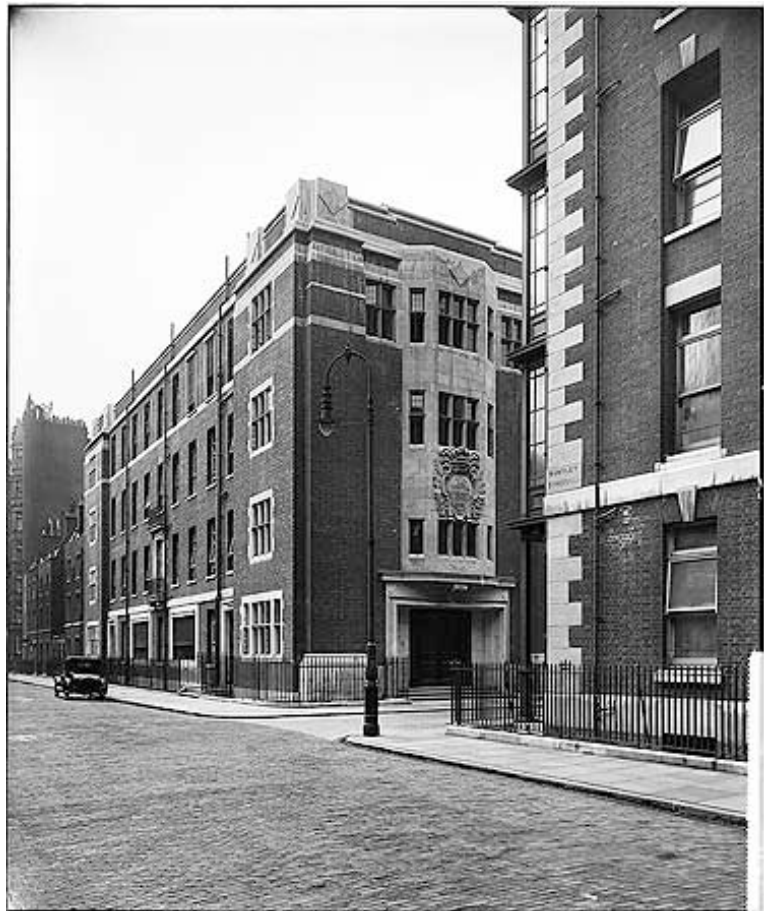
Figure 1: The newly constructed Royal Ear Hospital in 1927 (© English Heritage)
