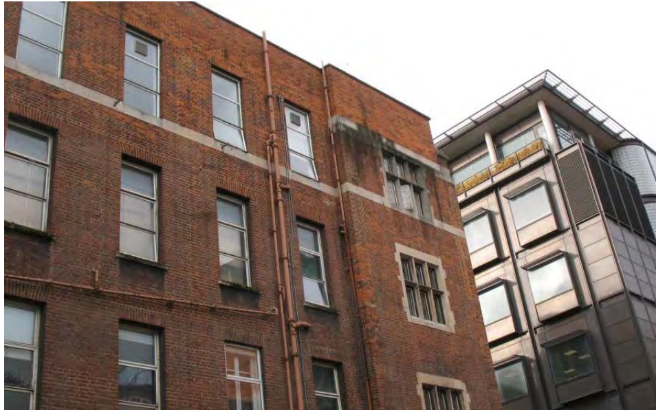
Image 11: Huntley St elevation. Evidence of water staining and local brick repairs on Copper St return. (Cat 4)
