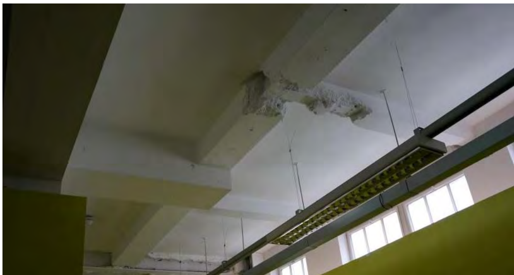
Image 4: Locally removed fire proofing of primary steel. (Cat 3)
