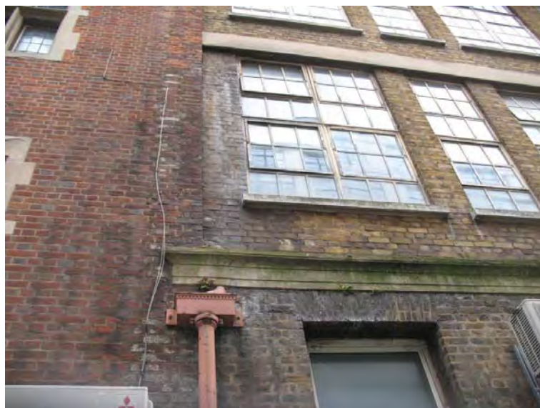
Image 21: Brick damage and possible local repairs (Cat 2)
