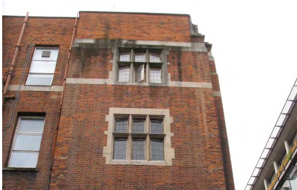
Image 13: Huntley St elevation. Evidence of water staining and local brick repairs on both corners of return. (Cat 4)
