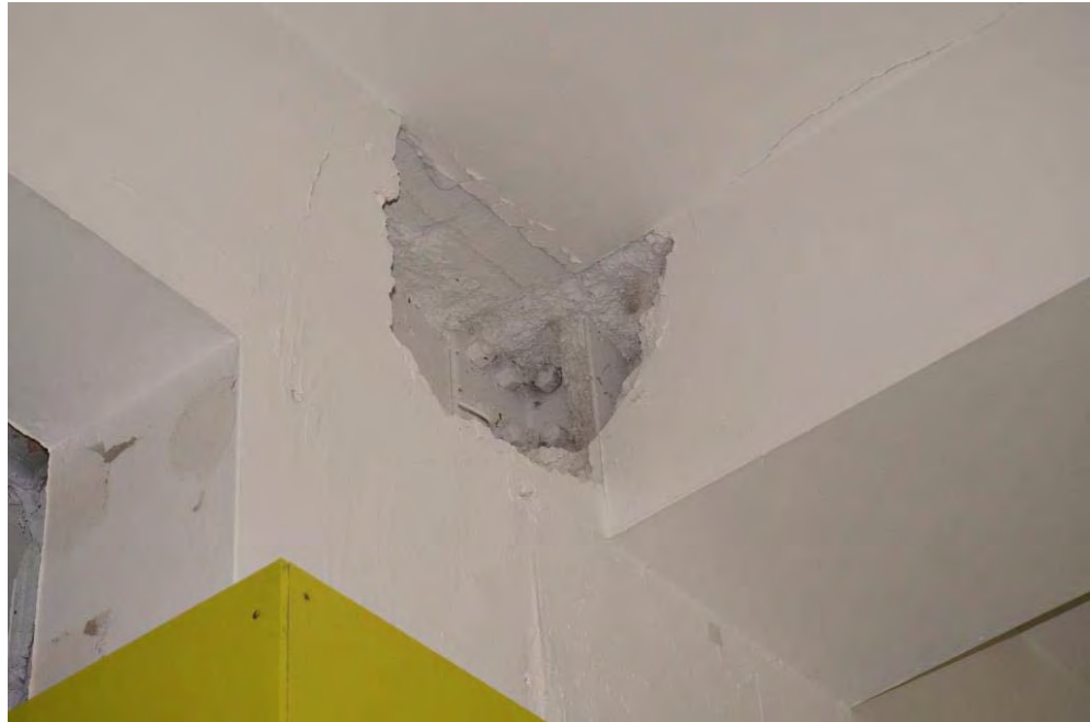
Image 7 Exposed steel beam to column connection. (Cat 3)
