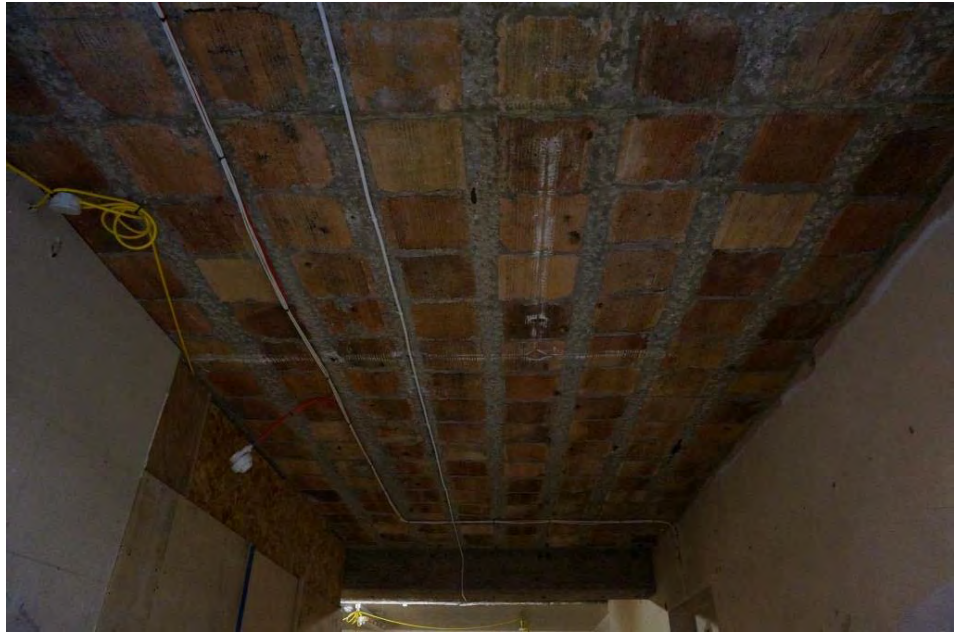
Image 1: Typical hollow-pot floor structure of building. Taken at underside of ground floor.
