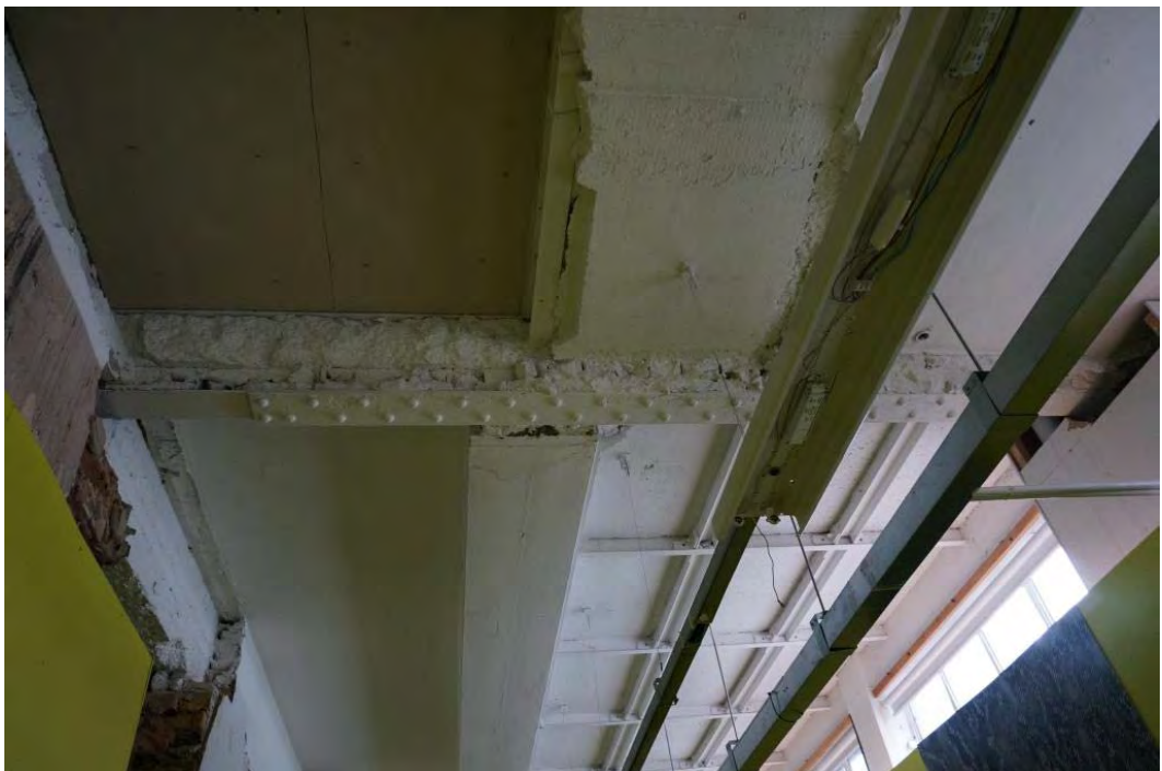
Image 6: Exposed steel grider beam with fire proofing cladding removed (Cat 3)
