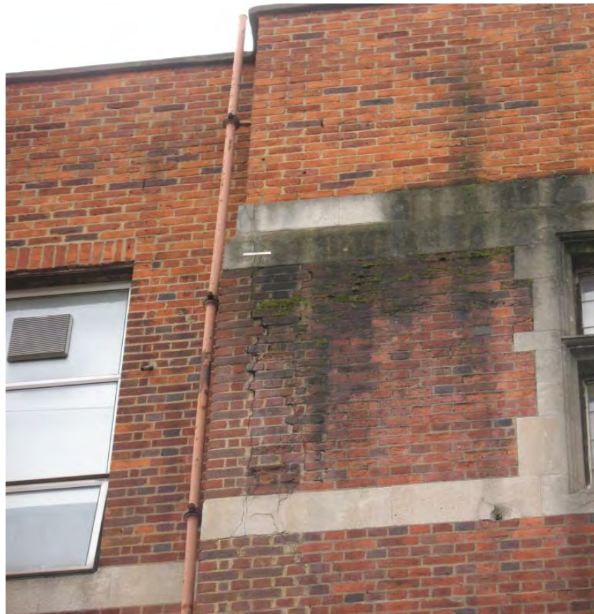
Image 12: Huntley St elevation. Significant defects in brick façade and visible water damage. Cracking of brick façade and bowing of damaged brick potentially caused by deterioration and likely delamination of steel support structure of façade. (Cat 1)
