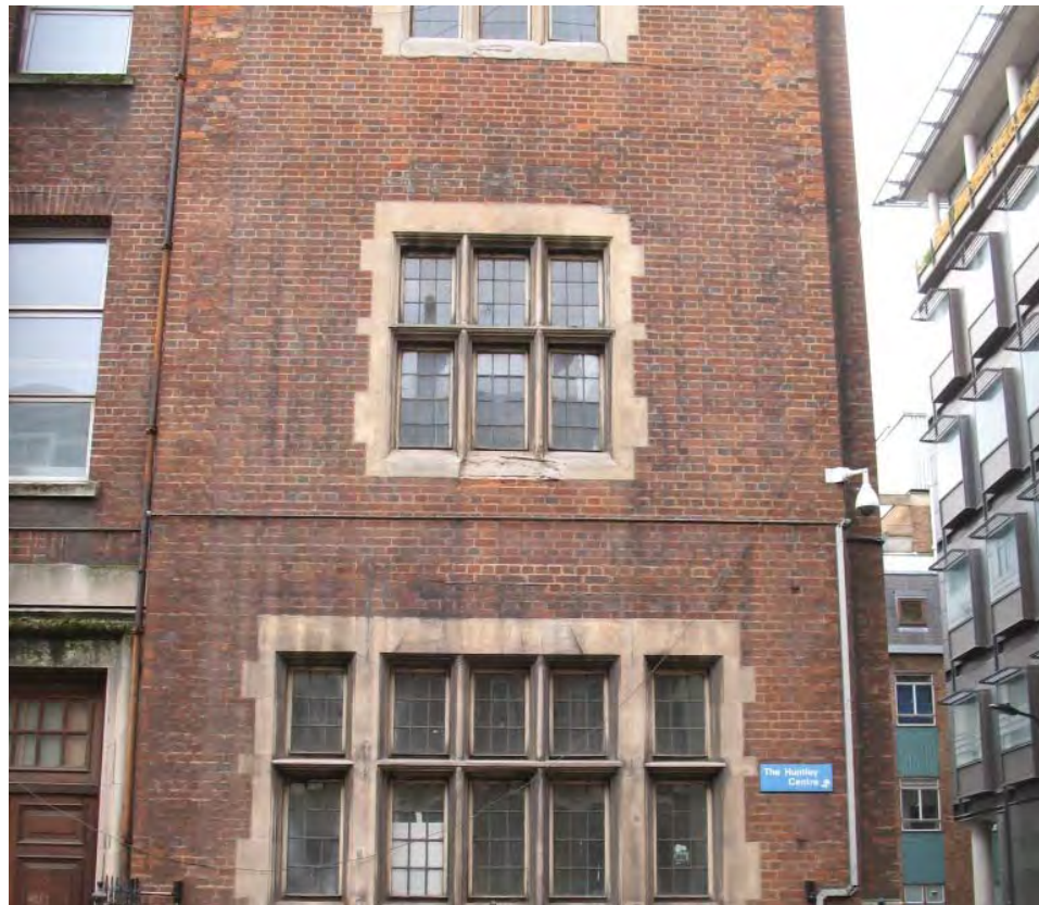
Image 14: Huntley St elevation. Evidence of water staining and local brick repairs on both corners of return. (Cat 4)
