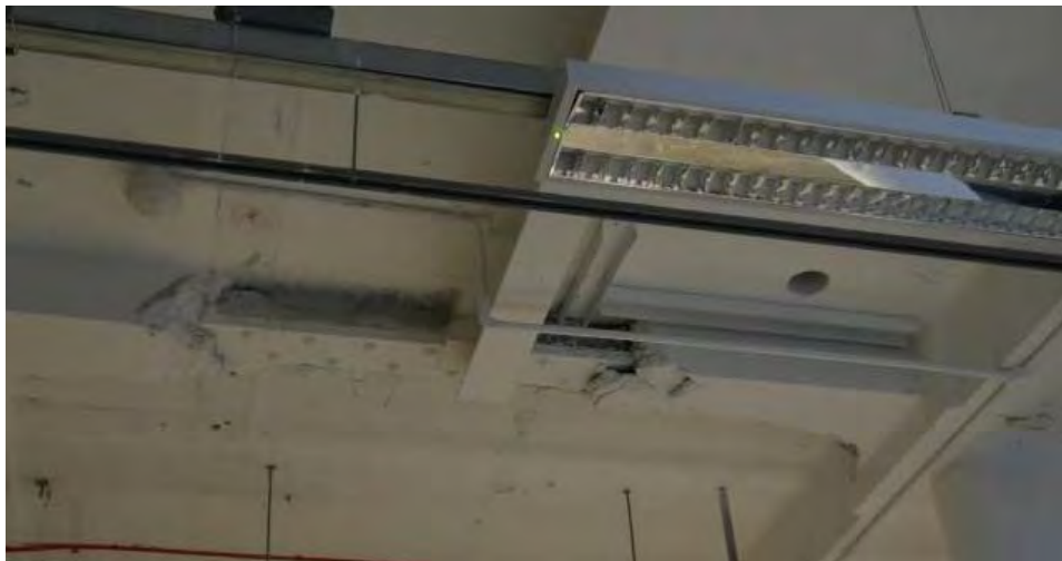
Image 2: Typical exposed steel girder beam, supporting floor structure. (Cat 3)
