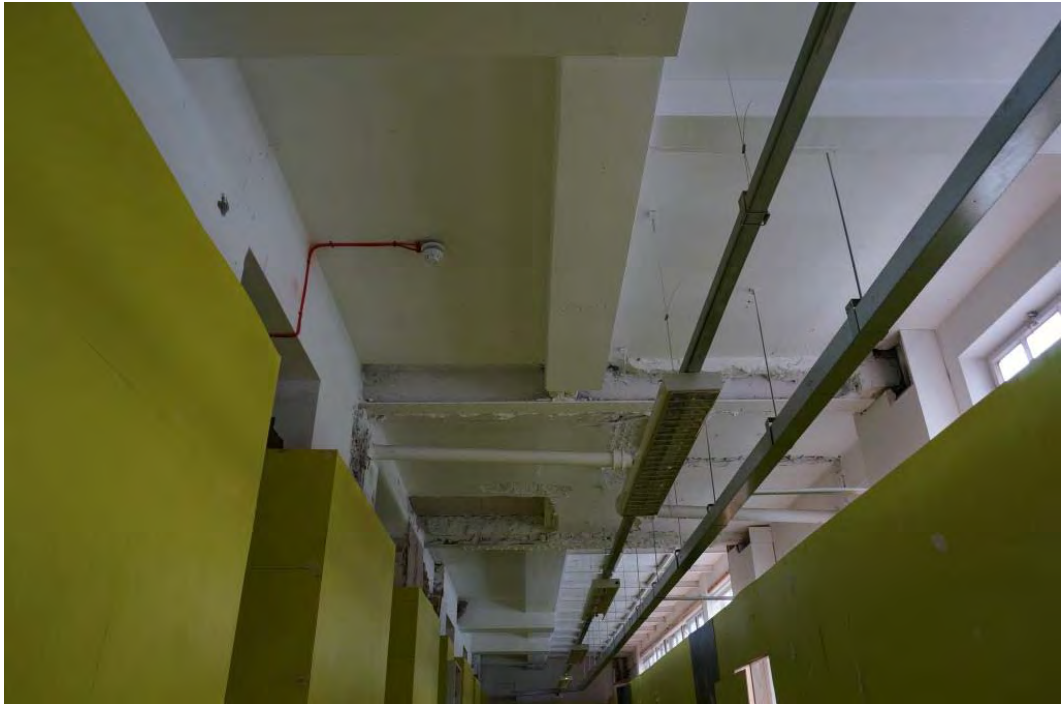
Image 5: Exposed primary steel structure (Cat 3)
