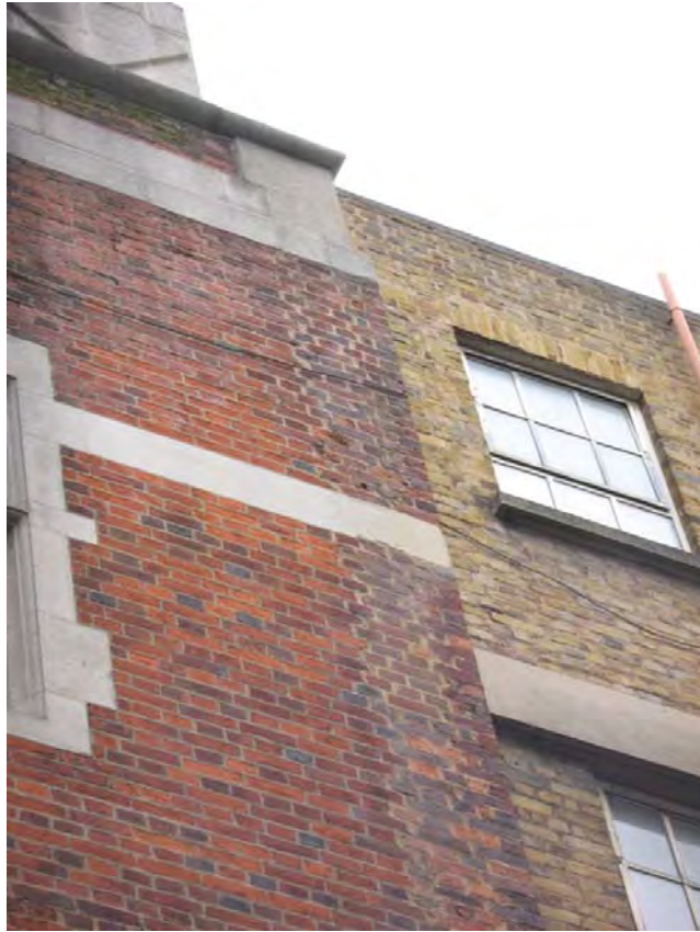
Image 20: Brick damage and possible local repairs (Cat 2)
