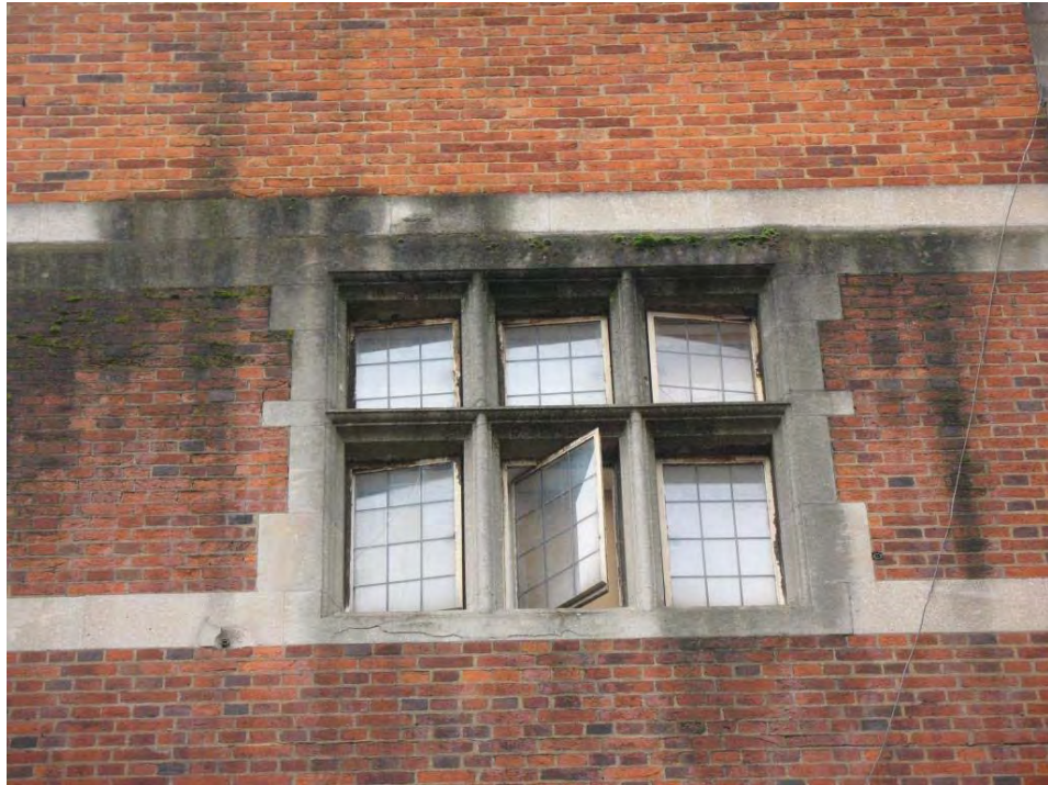
Image 15: Magnification of Image 13. Evidence of significant water damage. Possible spalling of concrete window sill and cracking of brick work. (Cat2/3)
