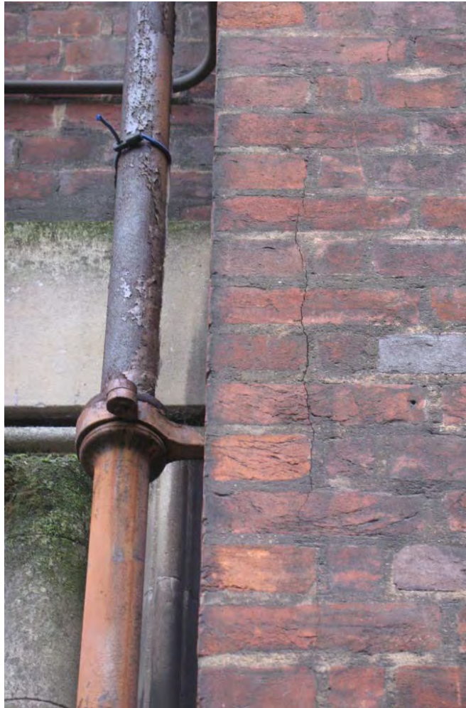
Image 18: Cracking in brick façade likely due to water ingress. (Cat 2)
