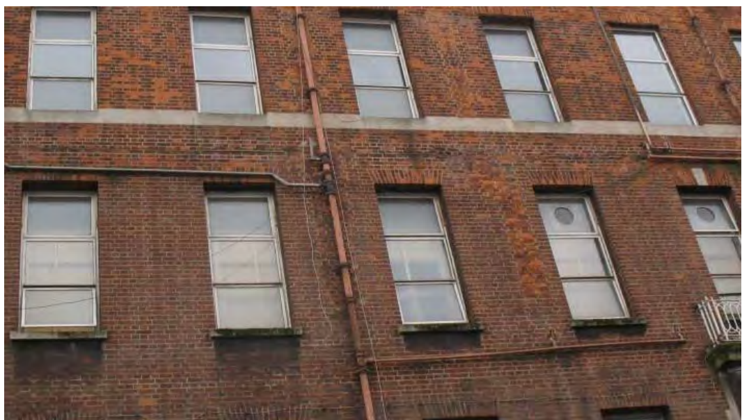
Image 10: Huntley St elevation. Evidence of water staining and local brick repairs. Linear cracking in brick above 3rd floor windows. (Cat 2)
