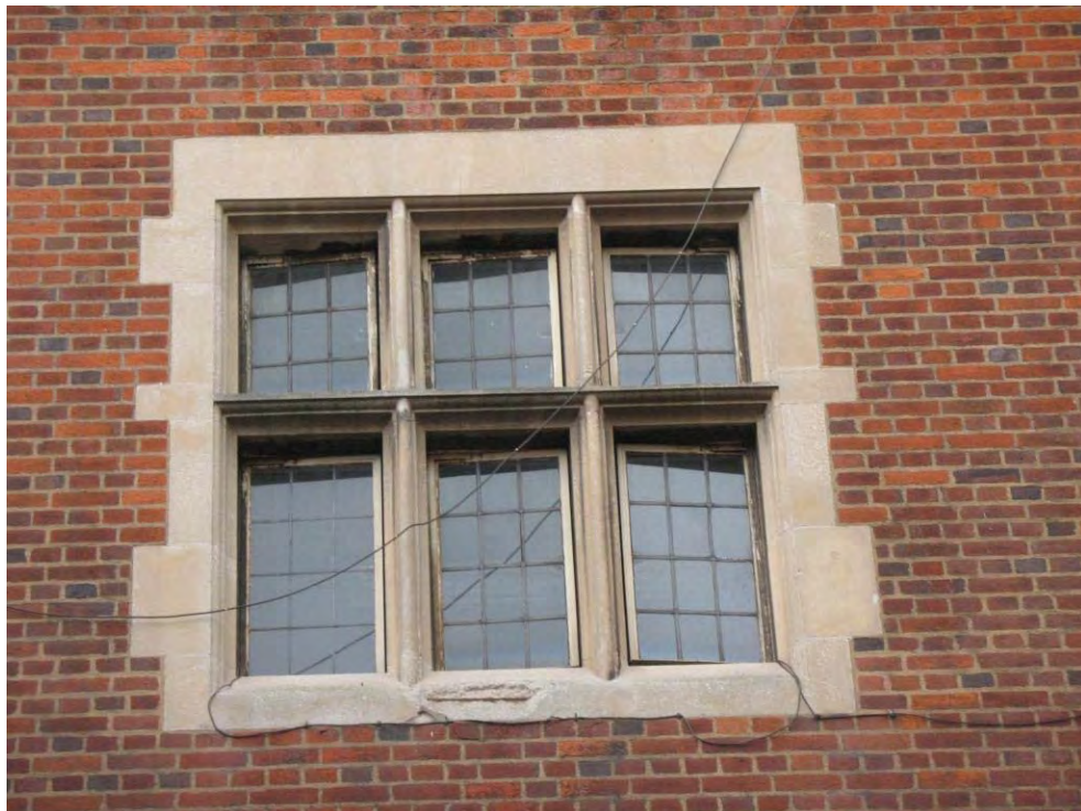
Image 16: Magnification of Image 14. Spalling of concrete window sill exposing reinforcement. (Cat 3)
