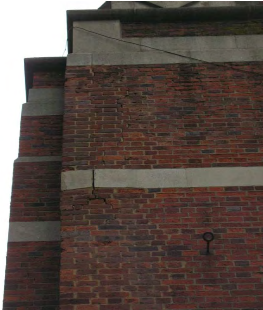
Image 19: Significant cracking and spalling brick and concrete. Likely deterioration of support structure with delamination of steel stansions forcing façade to crack and move. (Cat 1)
