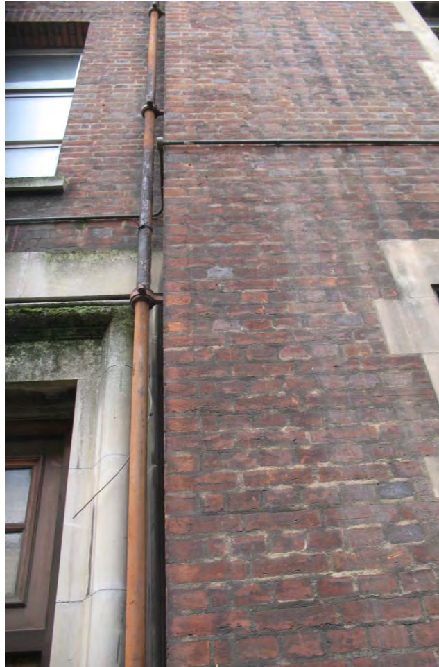
Image 17: Water effects along corner of façade return adjacent to downpipe. (Cat 4)
