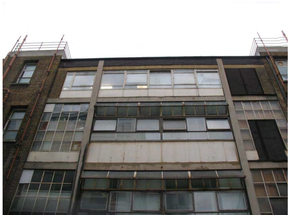
Image 8: External view of infill of original external balconies on Shropshire Place elevation
