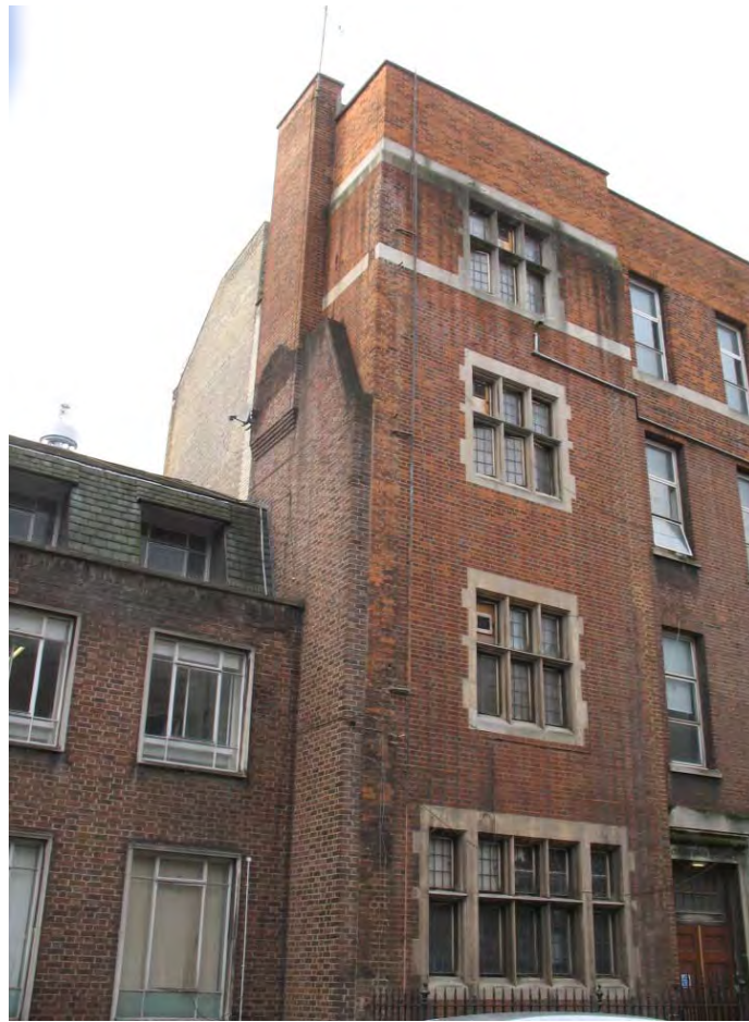
Image 9: Huntley St elevation. Evidence of water staining and local brick repairs. (Cat 4)
