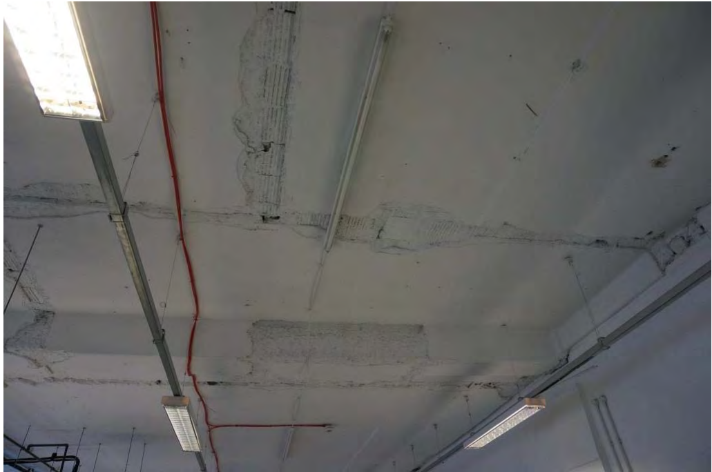
Image 3: Deterioration of finishes and fire proof cladding to structural elements. (Cat 3)
