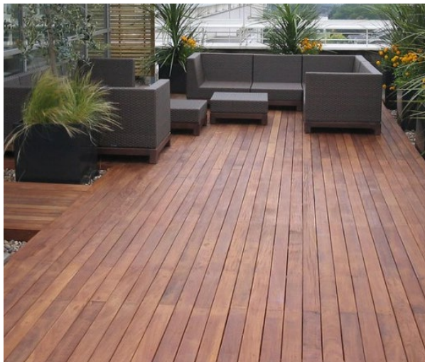
Hardwood decking to roof terrace
