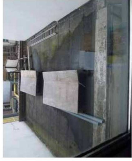
View from First floor window, looking south
