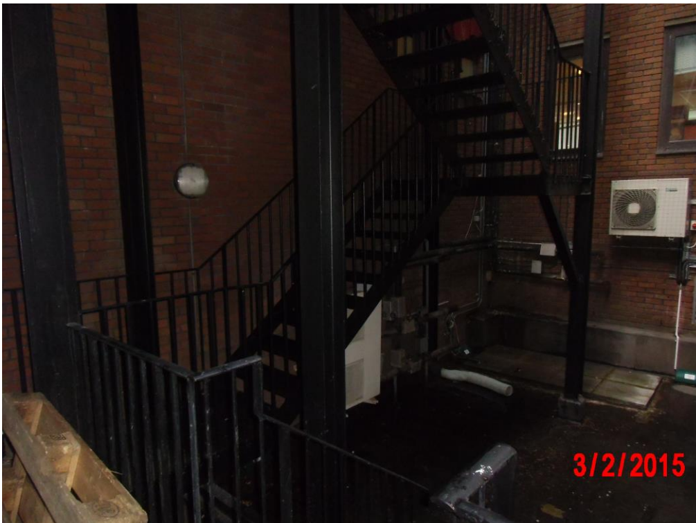
Area at Base of Lightwell
