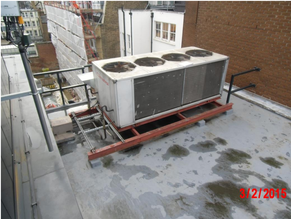
Existing Plant over Fourth Floor Plant Room
