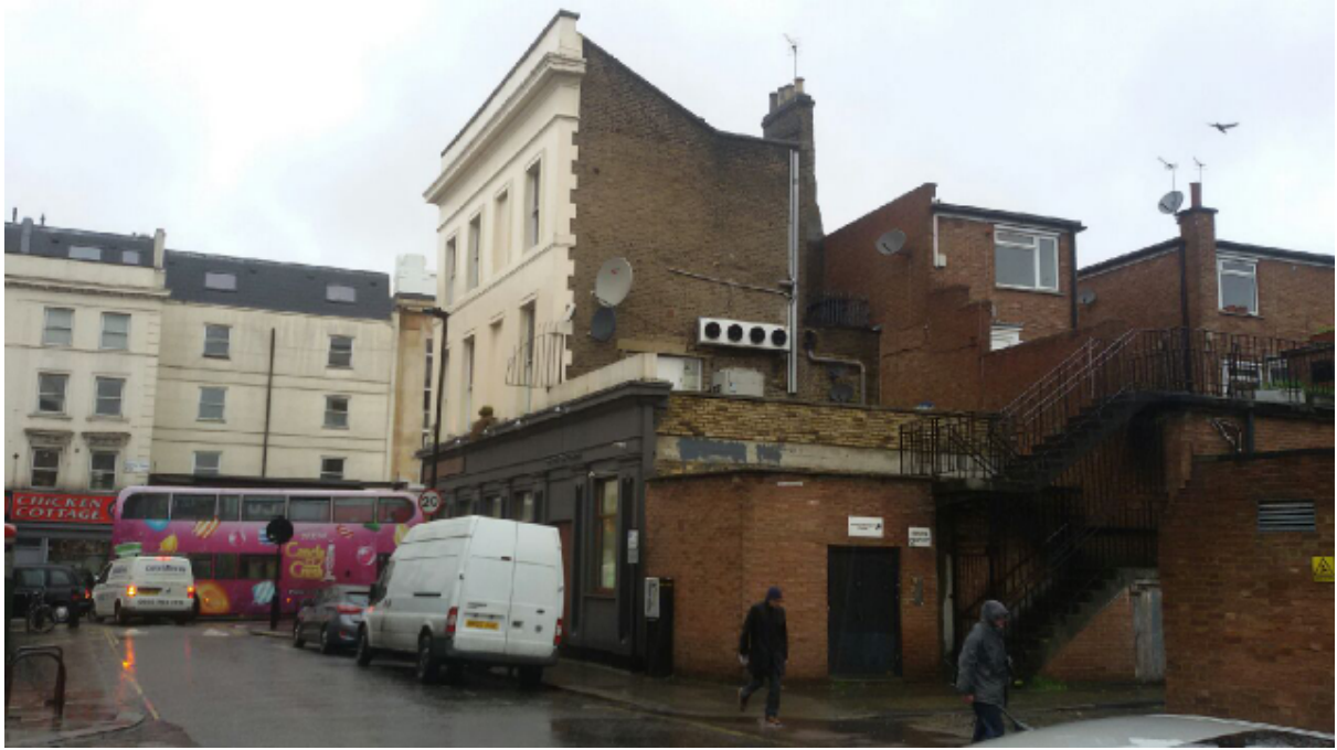
Side and rear of site from Patshull Road
