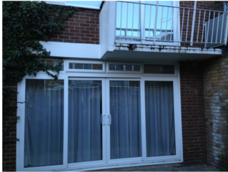
Photo showing existing rear elevation of No. 29
