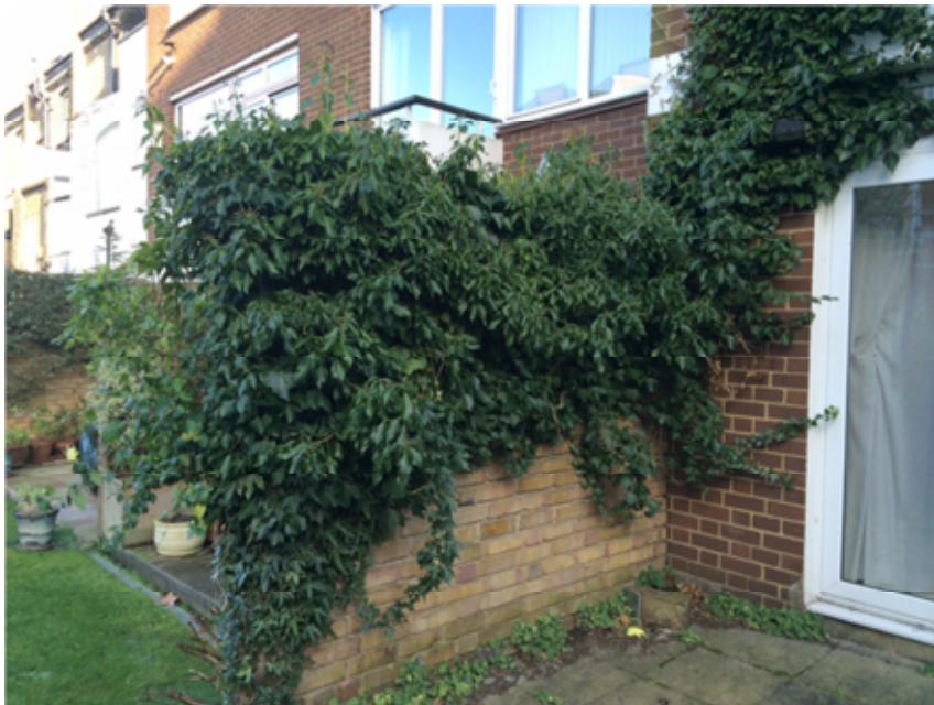
Photo showing existing boundary wall between No. 28 and No. 29
