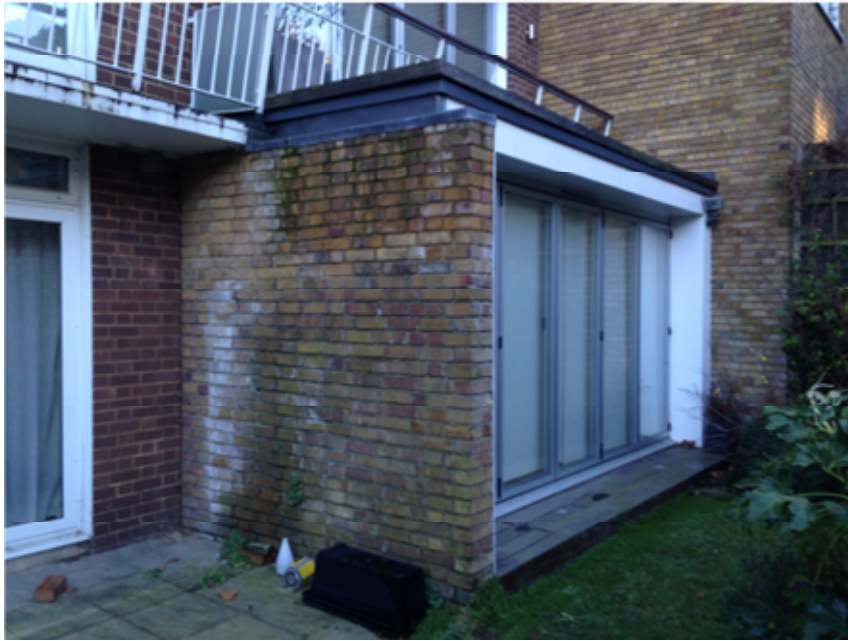
Photo showing ground floor extension at the rear of No. 30
