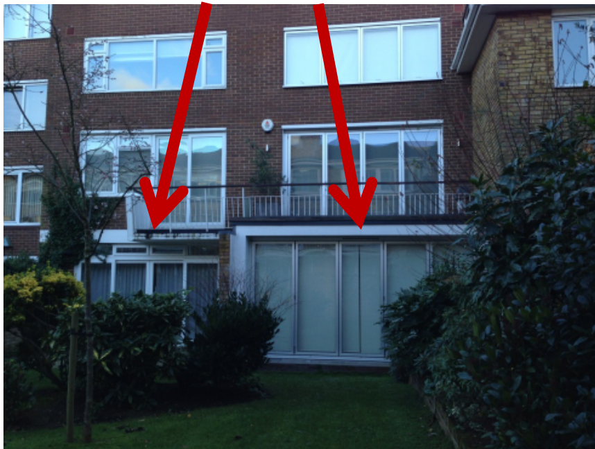
Photo showing rear elevation of No. 29 and No. 30
