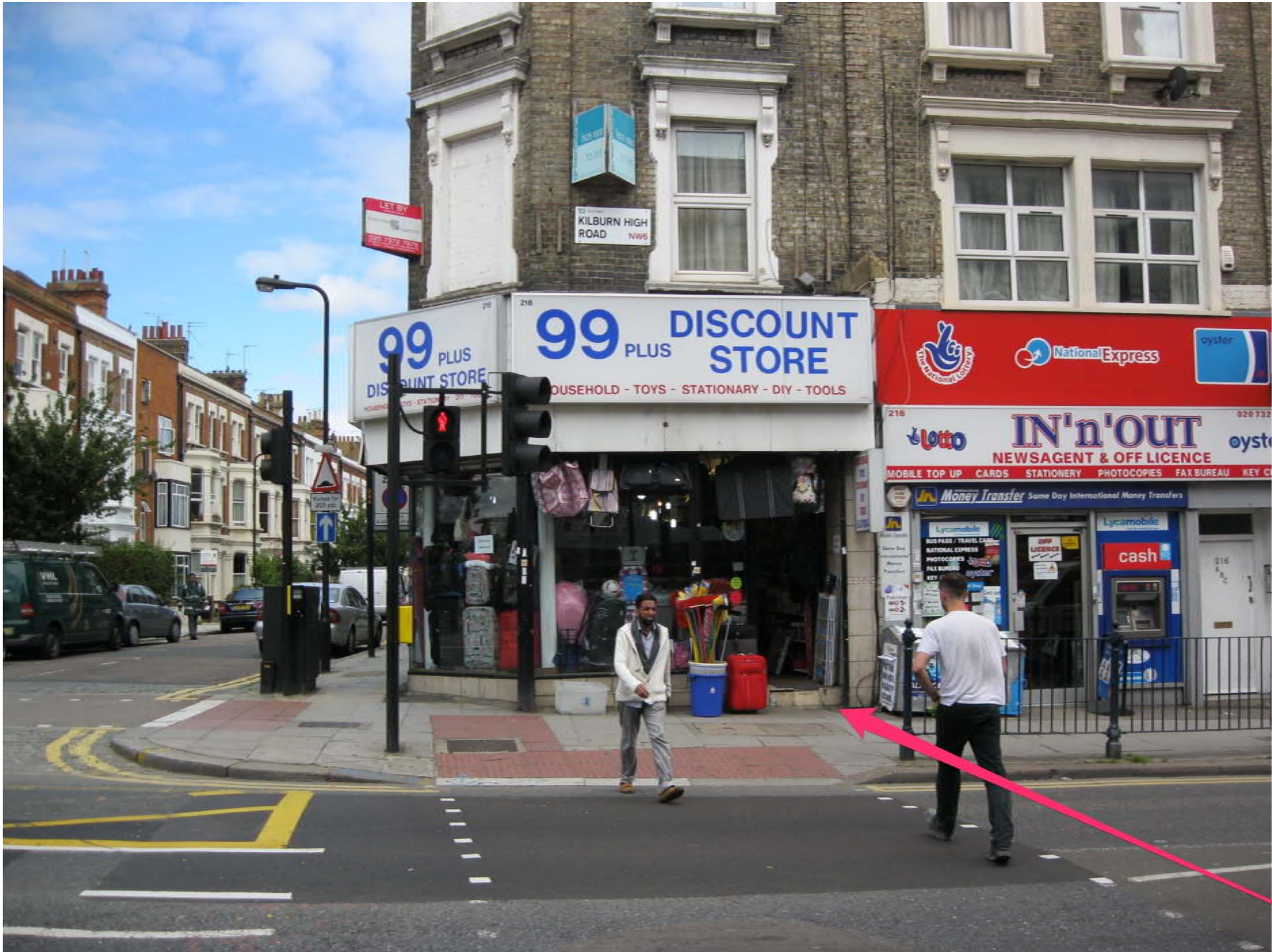
The existing entrance is not ramped
