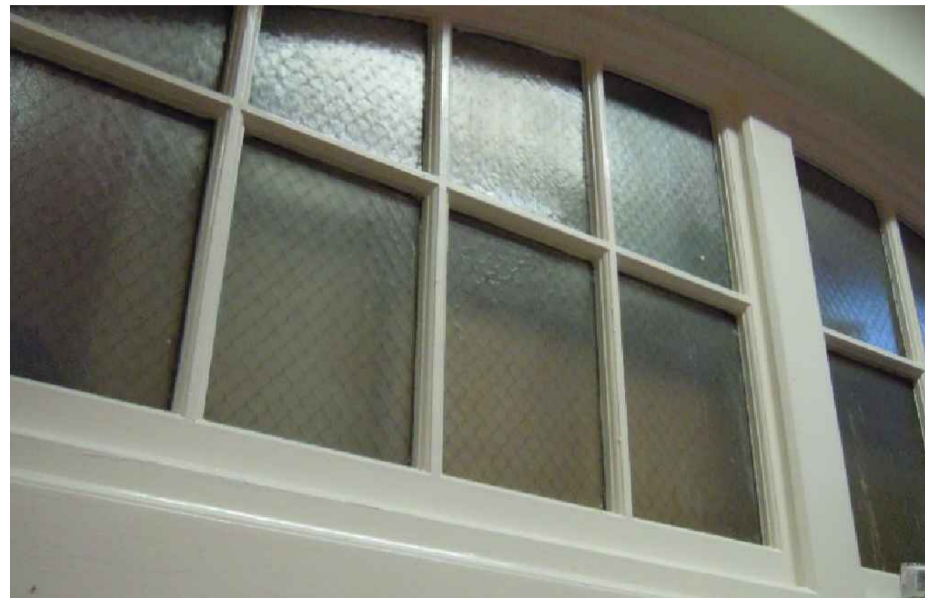
FIRST FLOOR WEST - HALL WCS
