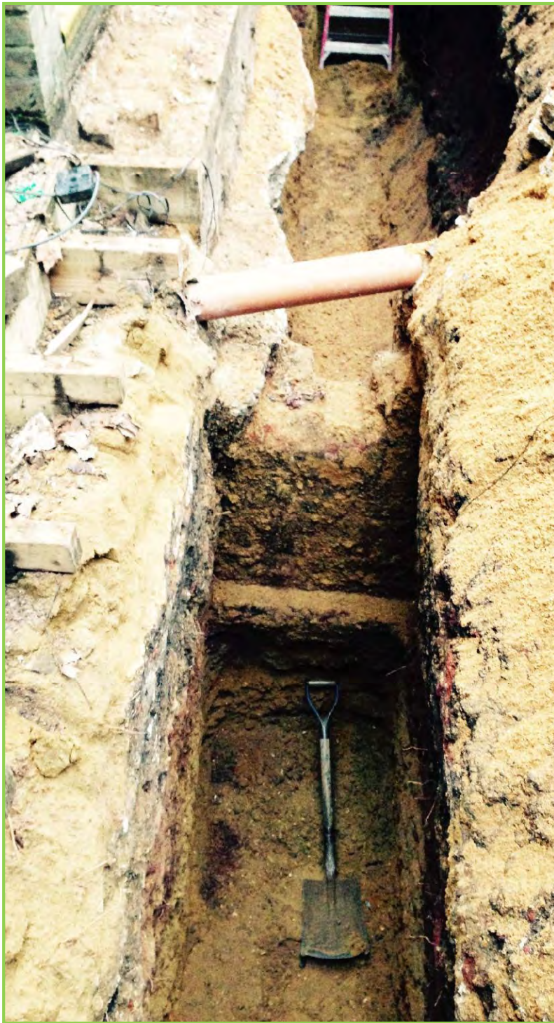
Trench bottomed out at 2.6m below rear garden level
