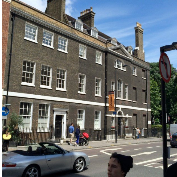
Figure 7: To the left hand side of the image the section of the building that used to be joined to No. 6 Bloomsbury Square until c.1880.
