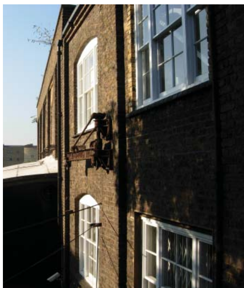
Existing windows - Arched and straight head on existing east elevation
