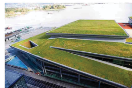
Extensive Green Roof
