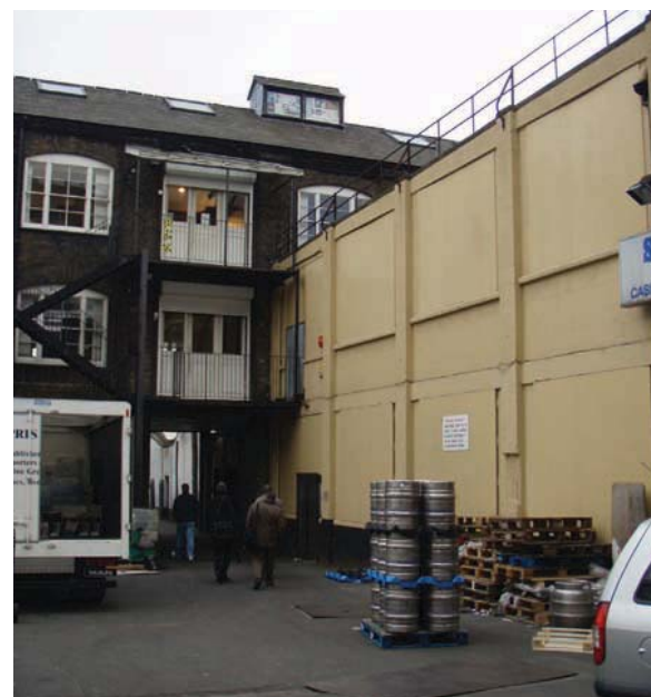
Painted Concrete Render and Steel Railings
