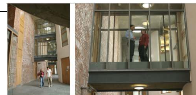
Contemporary glass and steel bridge link
