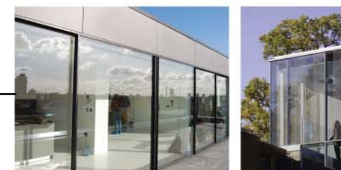
Glazed curtain wall
