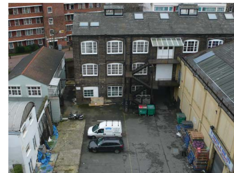
Existing view of courtyard
