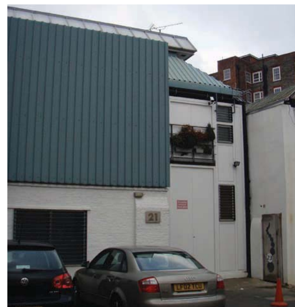
Corrugated Aluminium Cladding and Painted Brick
