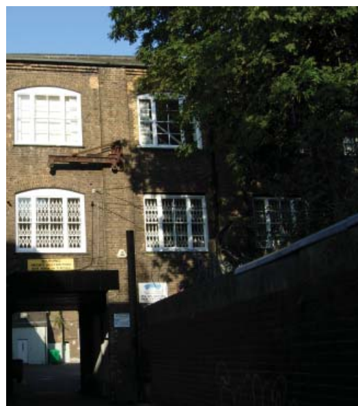
Existing windows - Arched and straight head on existing east elevation
