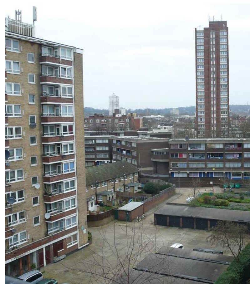
View of Hardington Tower on the left and Denton Tower on the right in the background.
