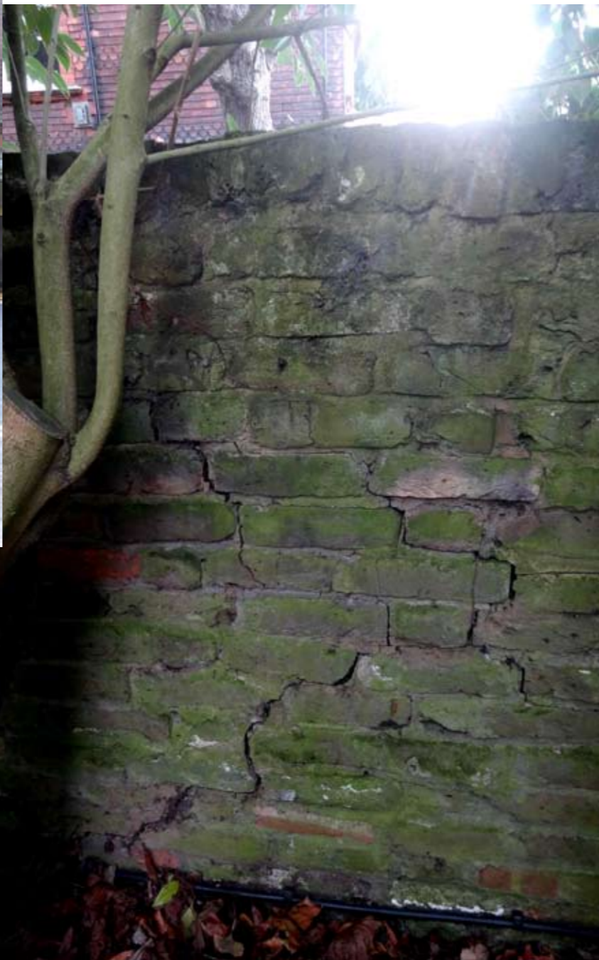
VIEW CRACKING FROM GARDEN SIDE
