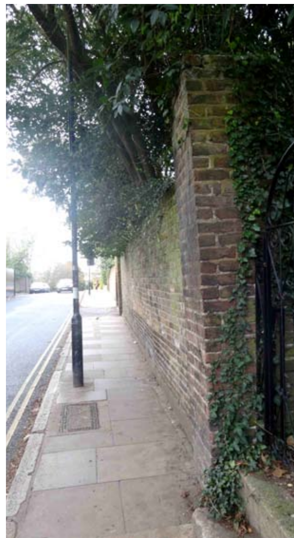
VIEW ALONG WALL FROM PEDESTRIAN GATE END
