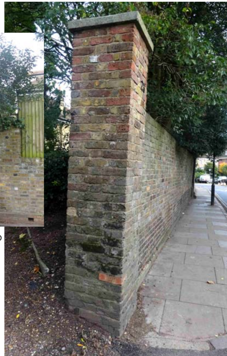
VIEW ALONG WALL FROM PILLAR AT VEHICLE ENTRANCE
