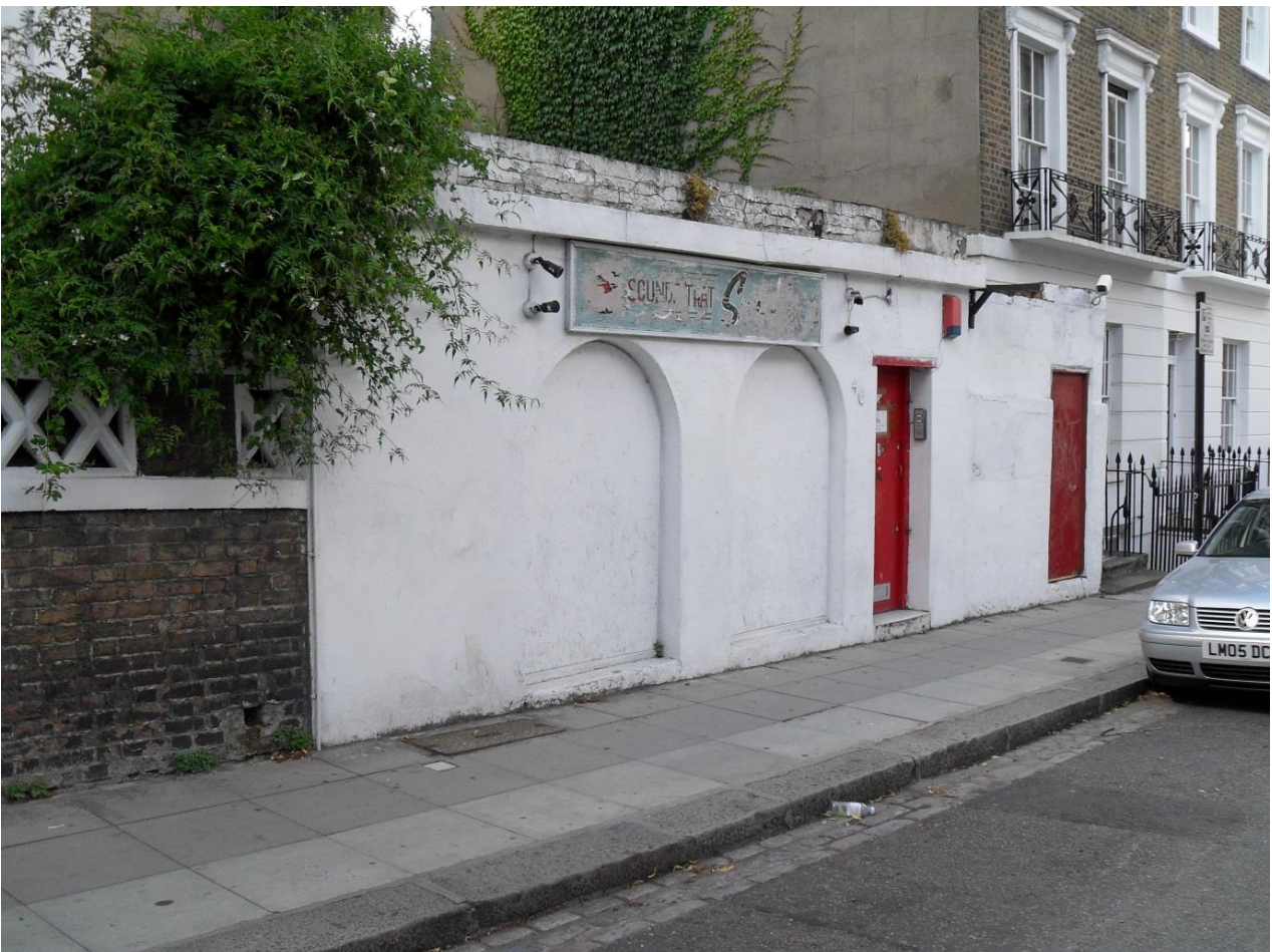
5.6 Close up view of No 46 Inverness Street, as existing
