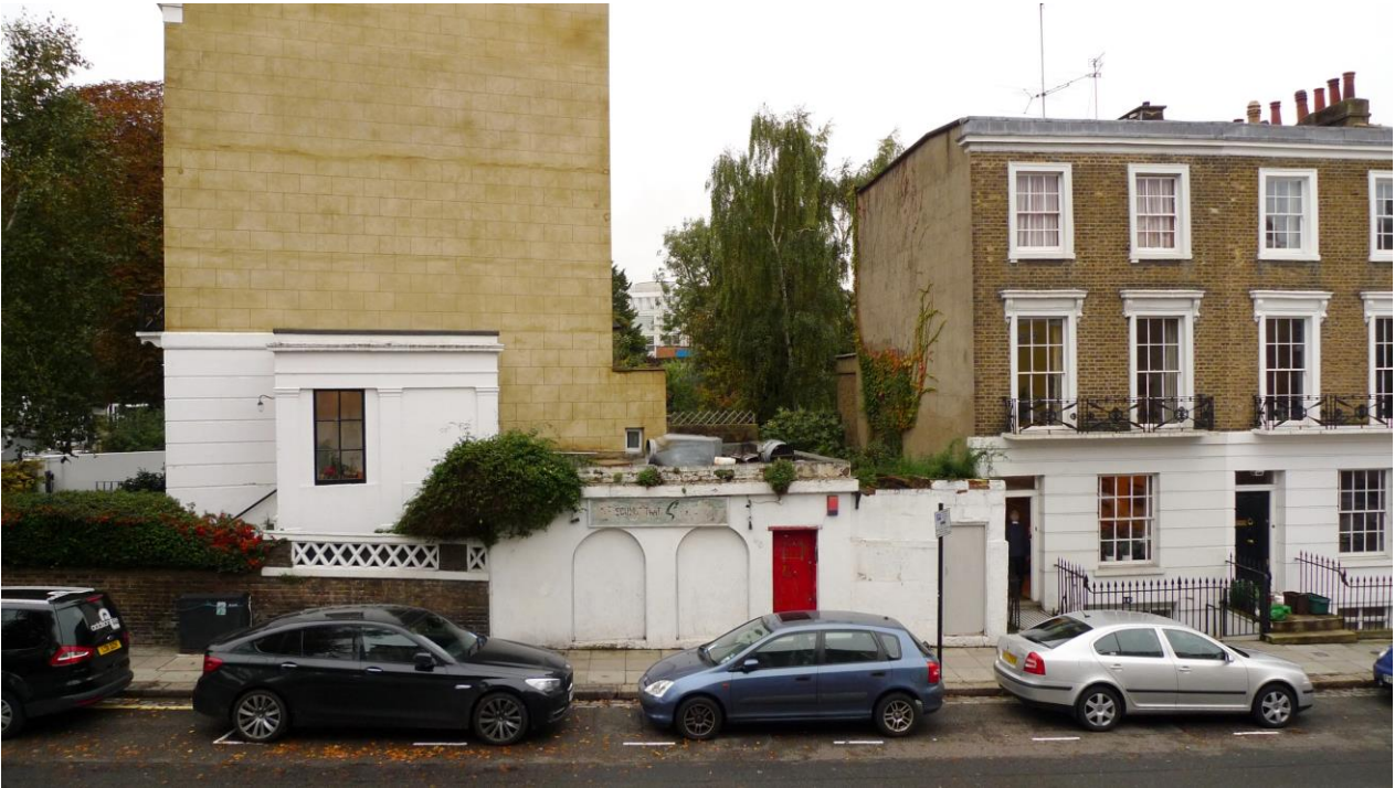
5.7 View of No 46 from first floor at No 43 Inverness Street, summer
