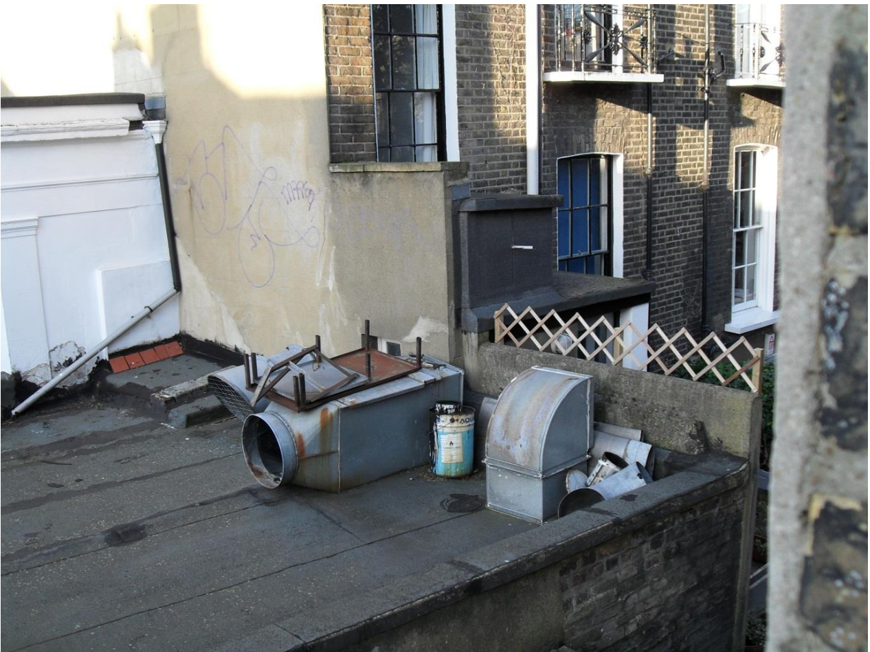
5.10 Existing roof to No 46 Inverness Street
