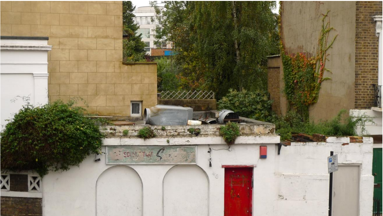
5.9 Close-up view of roof to No 46 Inverness Street
