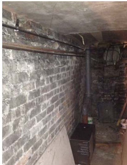
Figure 33 6 Sumatra road - existing cellar next to 4 Sumatra Road
