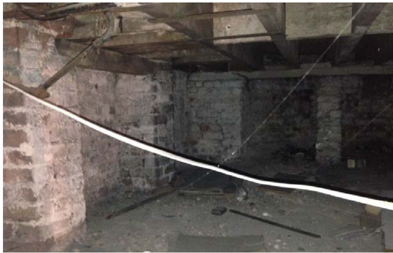
Figure 32 6 Sumatra road - existing cellar next to 8 Sumatra Road
