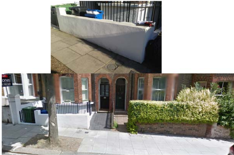
Figure 13 Slope - view front of the building
