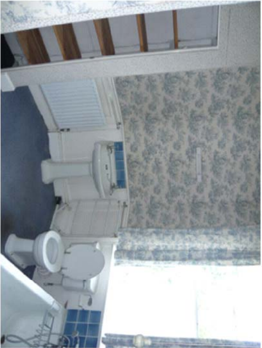
Overhaul and repair sash window. Repair and retain cornice. New bathroom stud wall partition shall have moulded plaster cornice and timber skirting to match the existing.
