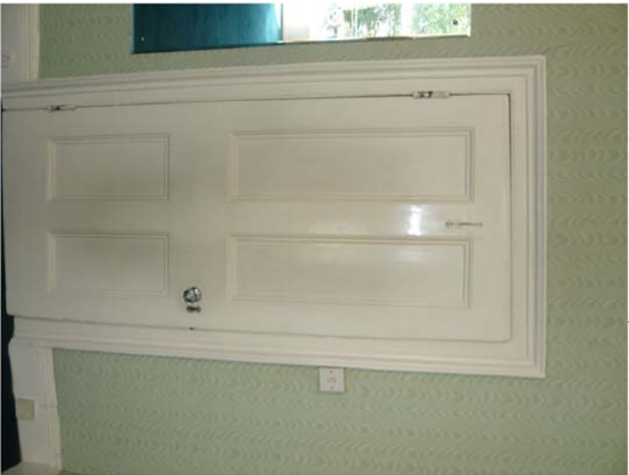
Strip and repaint timber door. Retain skirting and architrave. Remove cupb. door and retain door opening with architrave.
