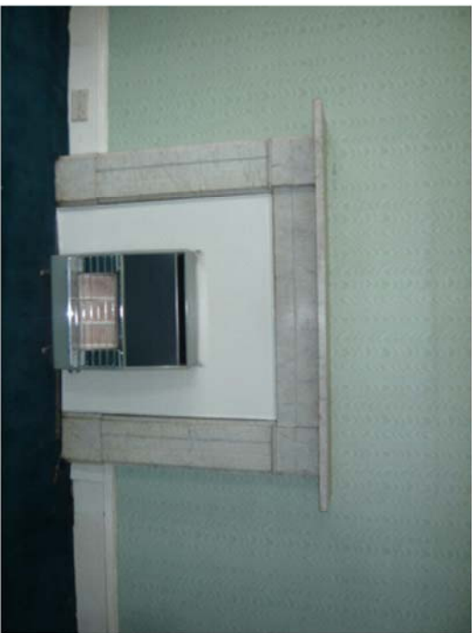
Existing fireplace surround to be retained. The fireplace and hearth to be reinstated.
