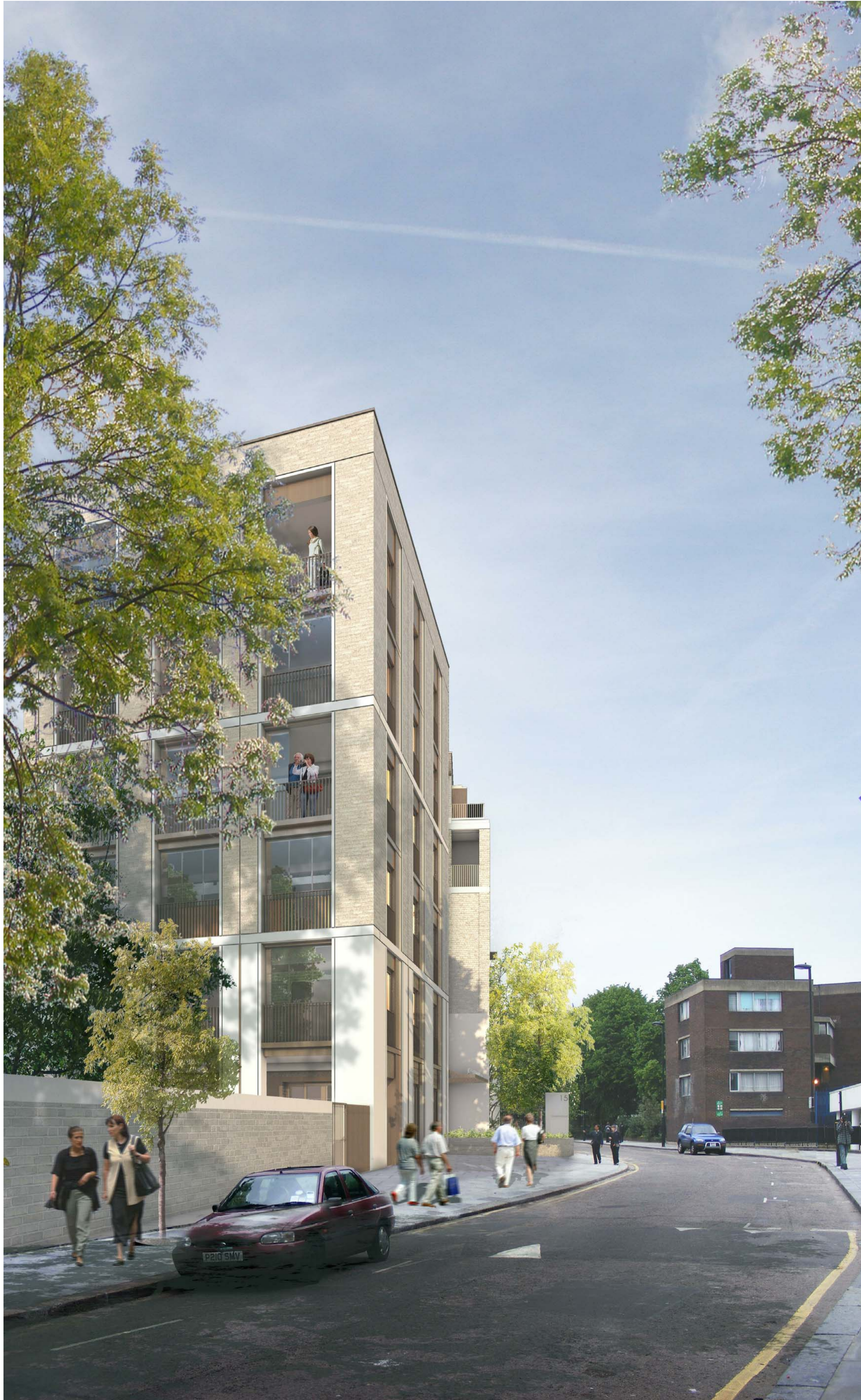
1. View North From Crogsland Road Towards Main Entrance
