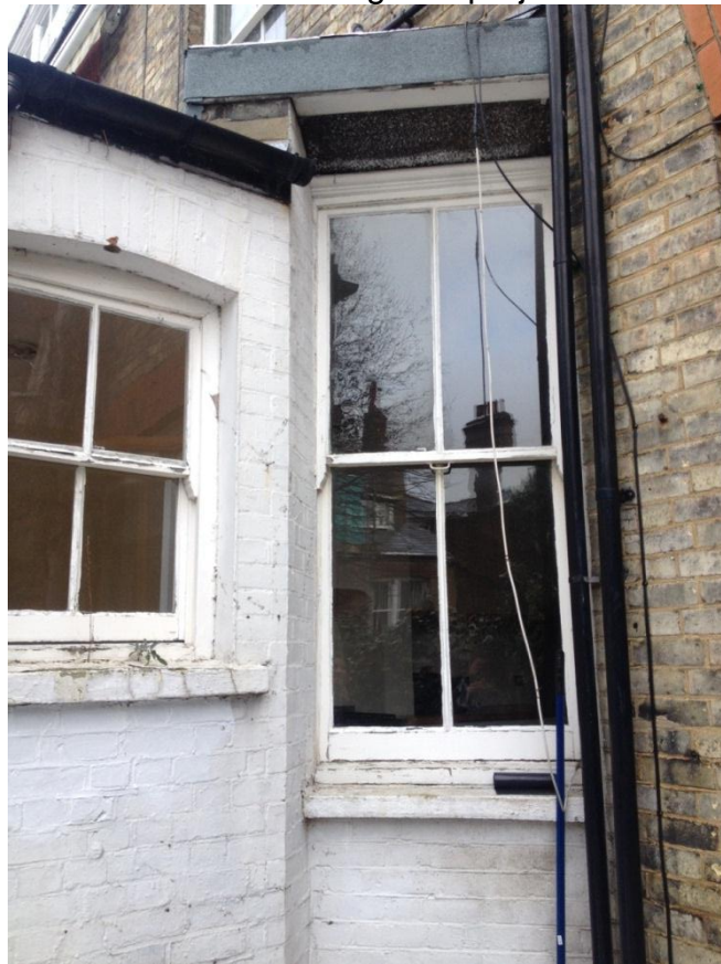
Photo 4- Existing windows in side elevation
