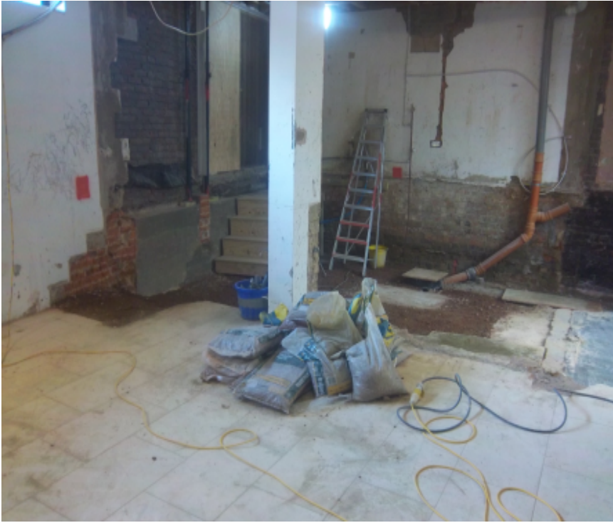
3. Ground floor level (internal)
