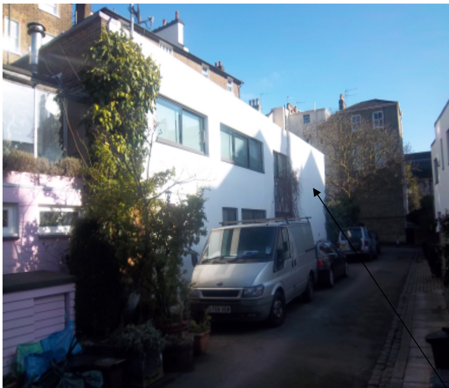
2. View of application property (no. 11) and elevation showing no existing windows
