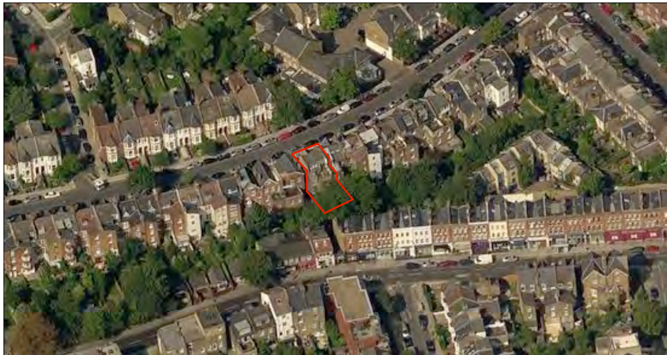
⑤ Aerial view of No. 76a Hillfield Road looking North
