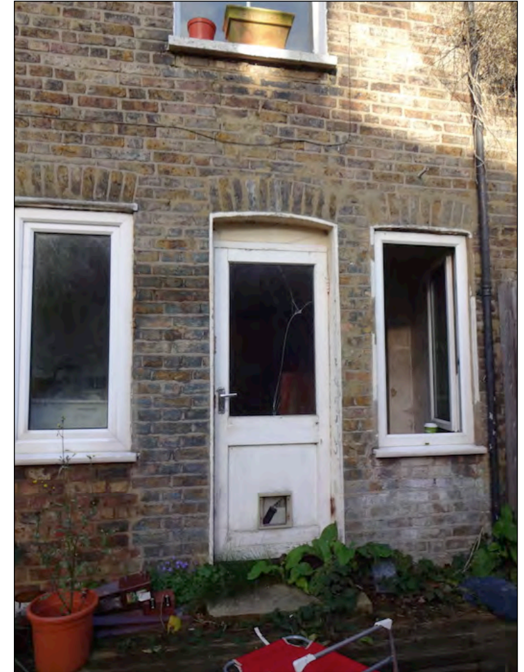
④ Existing rear elevation of 76a Hillfield Road
