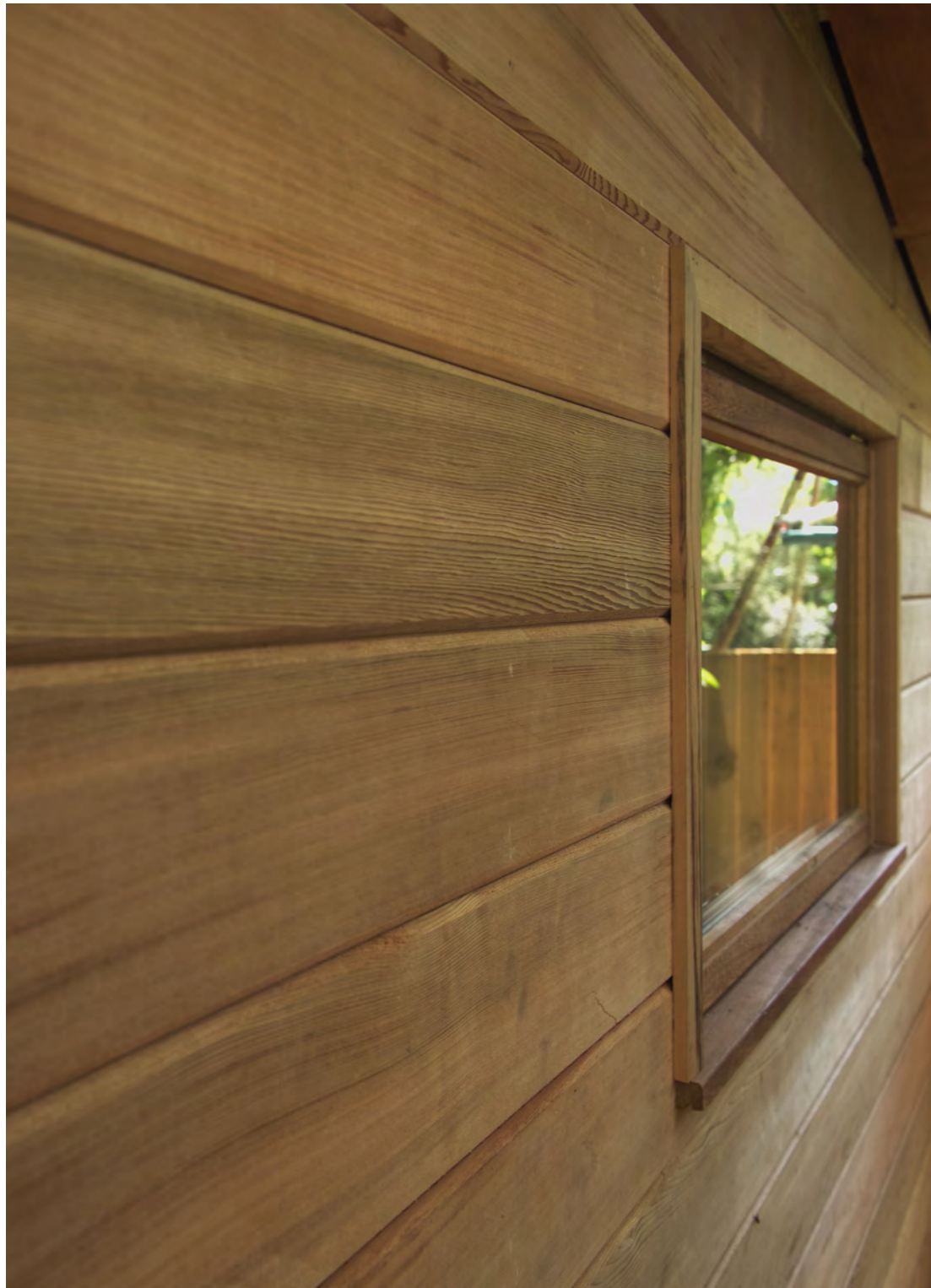
Western Red Cedar timber cladding
