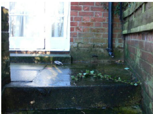
photo 4 flashing to no.9
