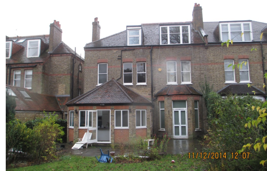
Figure 5 Rear Elevation of 55 Lancaster Grove
