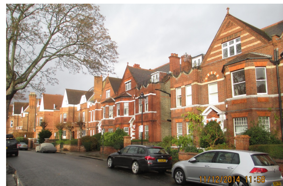
Figure 6 Lancaster Grove Looking East
