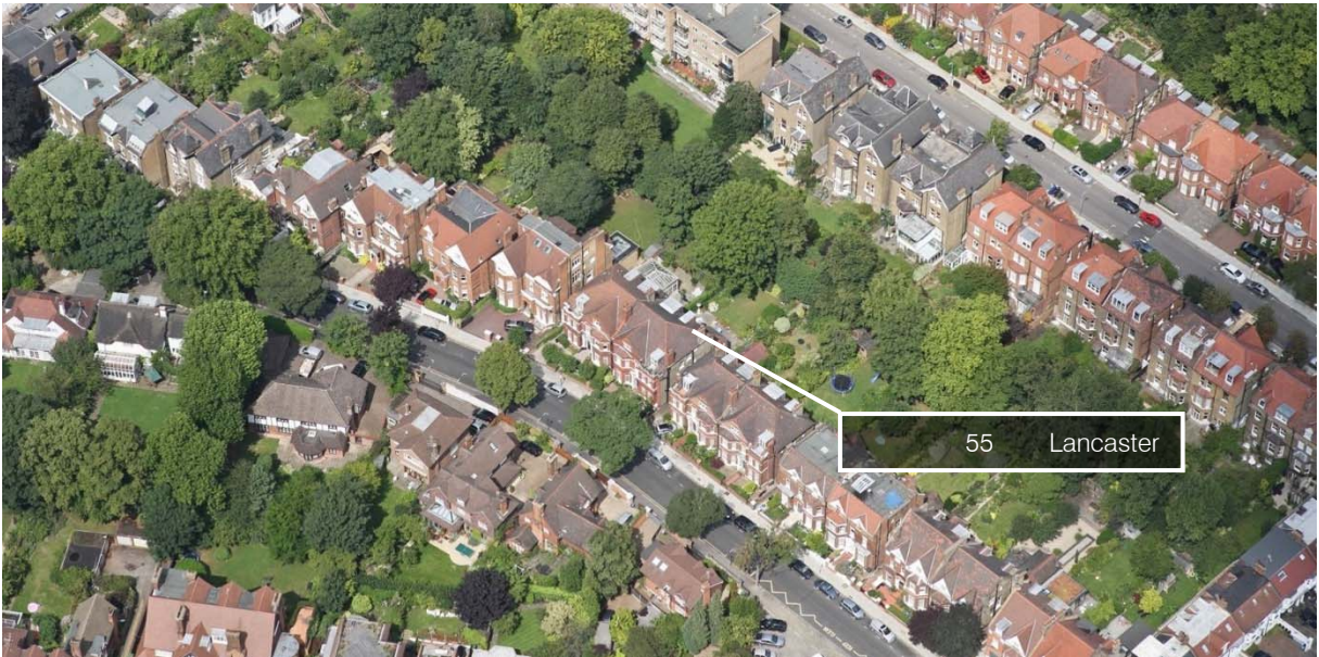
Figure 2 Aerial View of Site looking North
