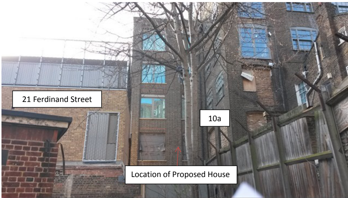
4. Application Site as Viewed from Electricity Sub-Station to North East
