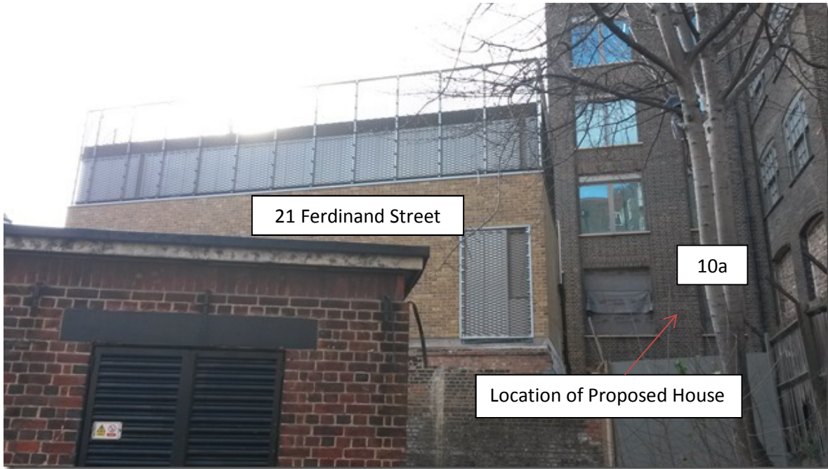
3. Application Site as Viewed from Electricity Sub-Station to North East
