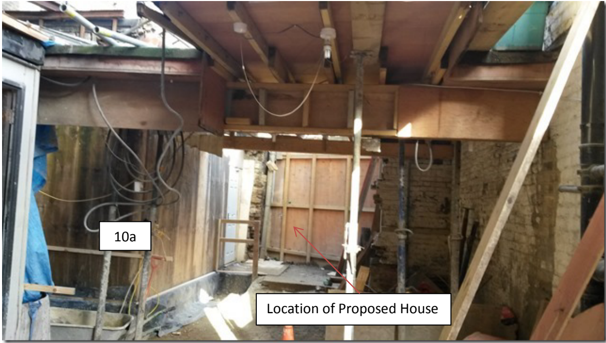
5. Application Site as Viewed from Rear Service Yard
