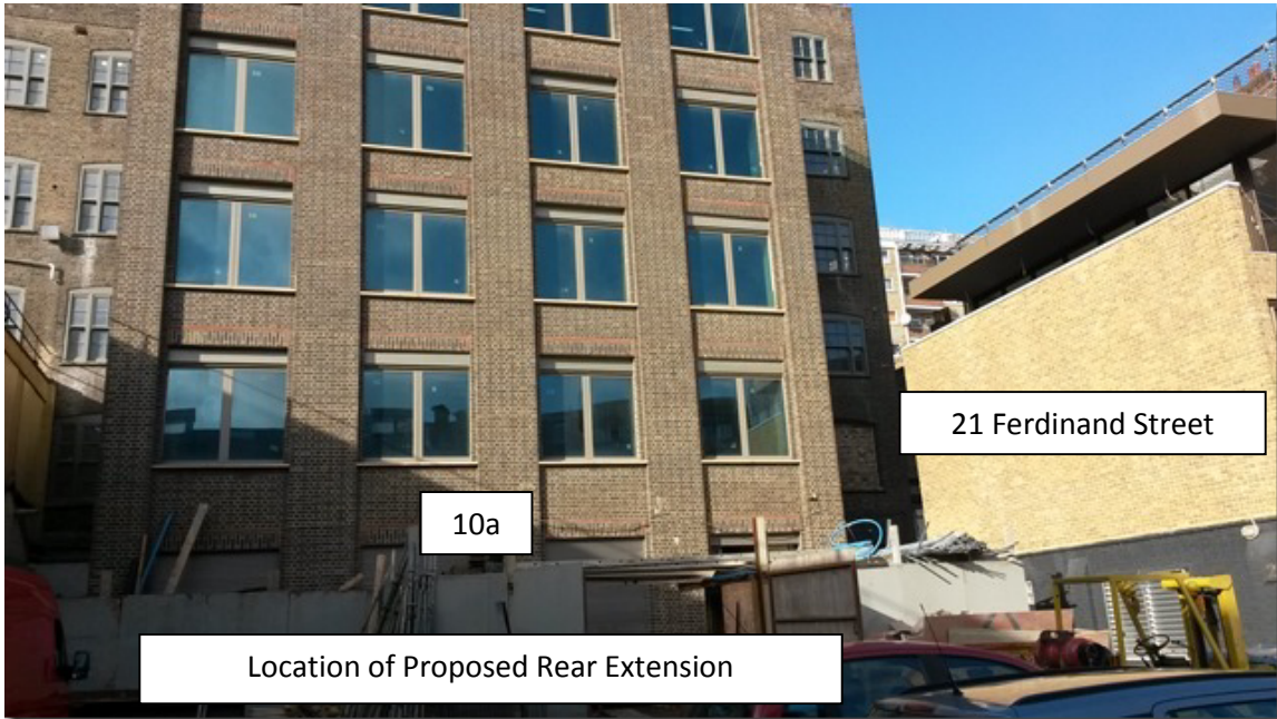
7. Rear Elevation of 10a as Viewed from Service Yard
