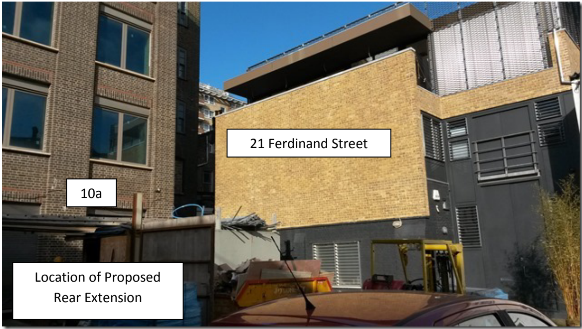
6. Rear Elevation of 10a as Viewed from Service Yard
