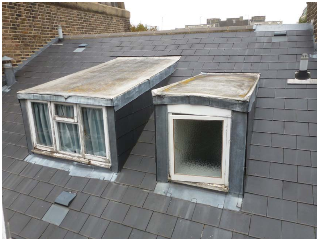
Photo 20: Taviton Annex - roof dormer windows.
