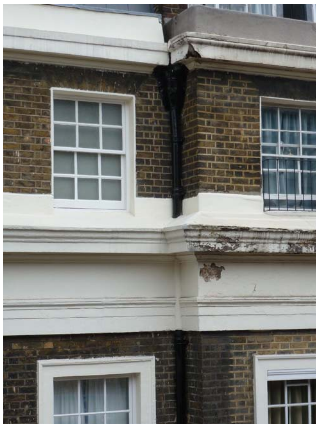
Photo 32: Taviton Annex - main cornice at neighbouring building.
