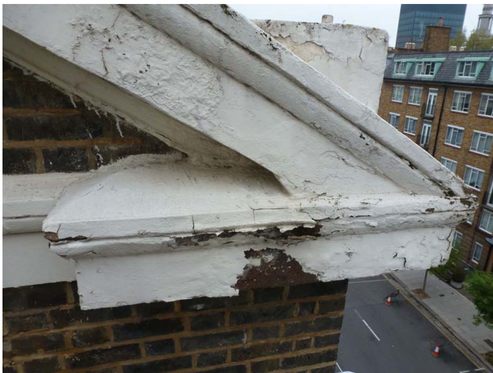
Photo 5: Endsleigh Street - gable end detail.
