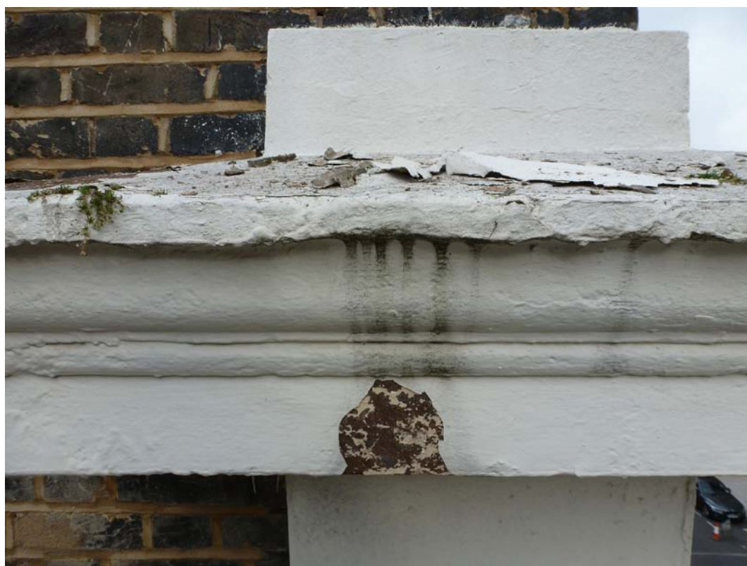
Photo 6: Endsleigh Street - main cornice band.
