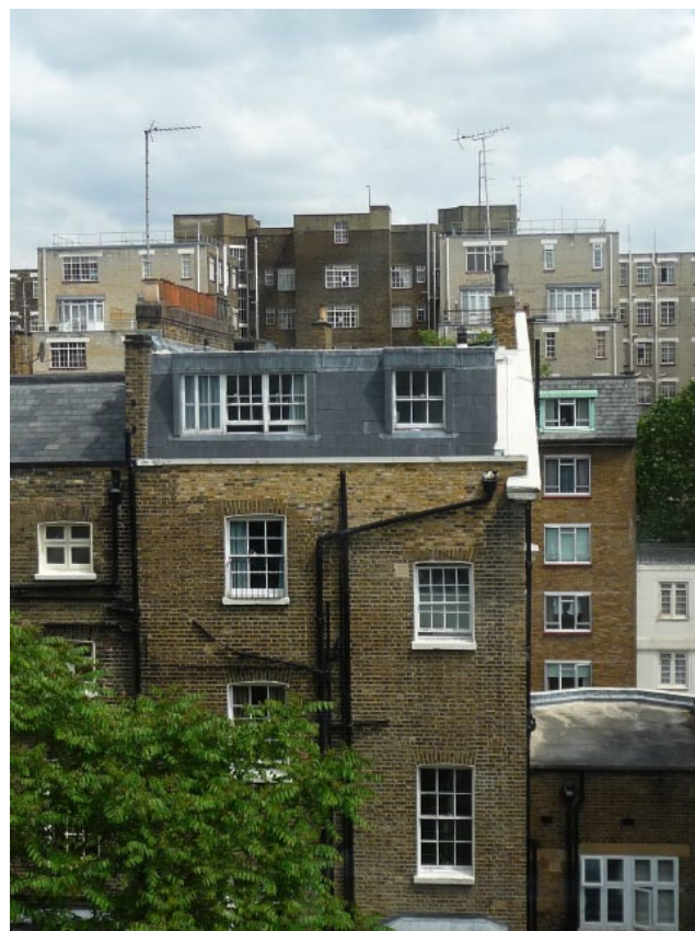
Photo 12: Endsleigh Annex: rear elevation
