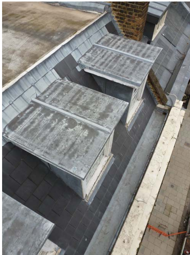
Photo 10: Endsleigh Street - roof dormers.
