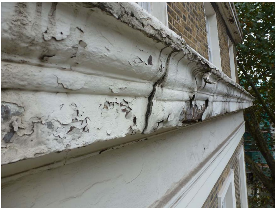
Photo 25: Taviton Annex - main cornice cill.
