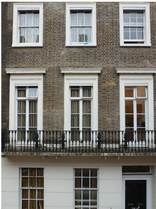
Photo 30: Taviton Annex - 1st floor balcony elevation.
