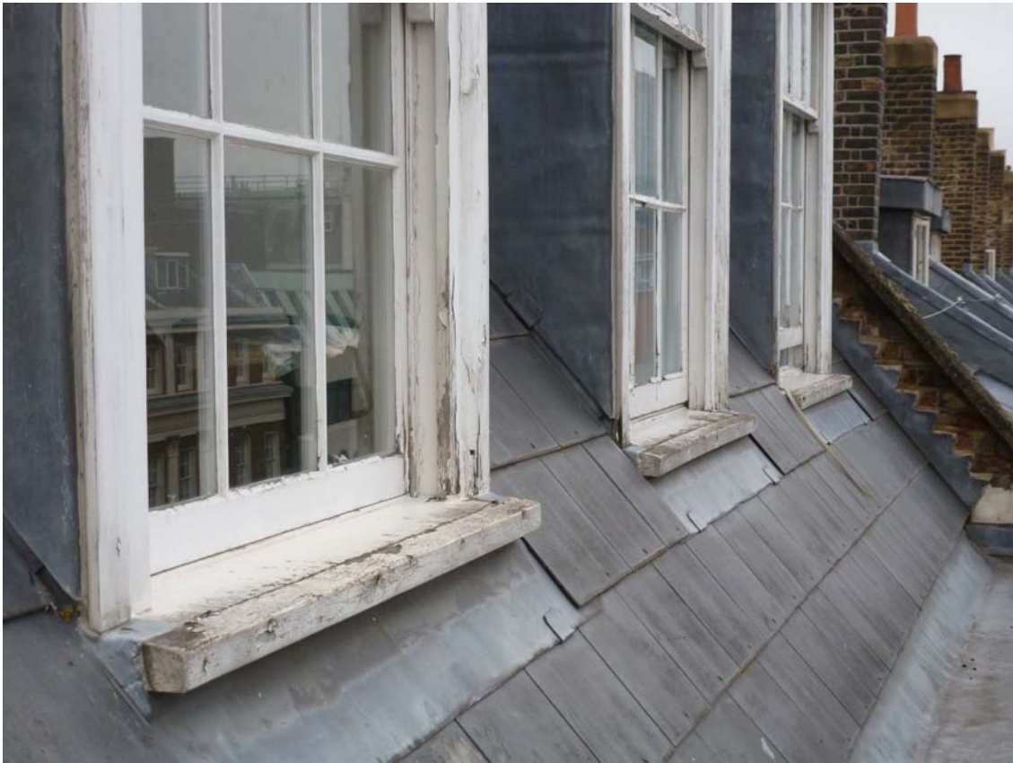
Photo 9: Endsleigh Street - front dormer windows as existing.
