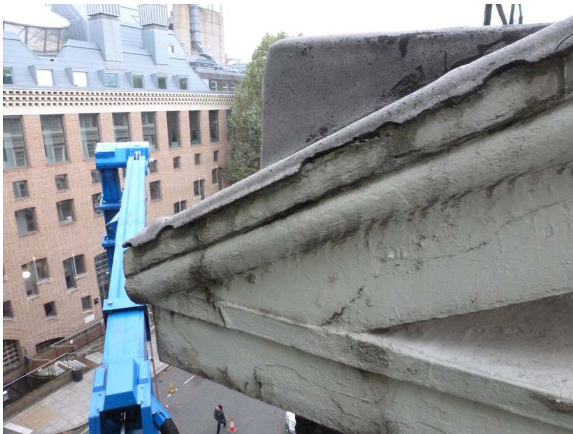
Photo 19: Taviton Annex - gable end.
