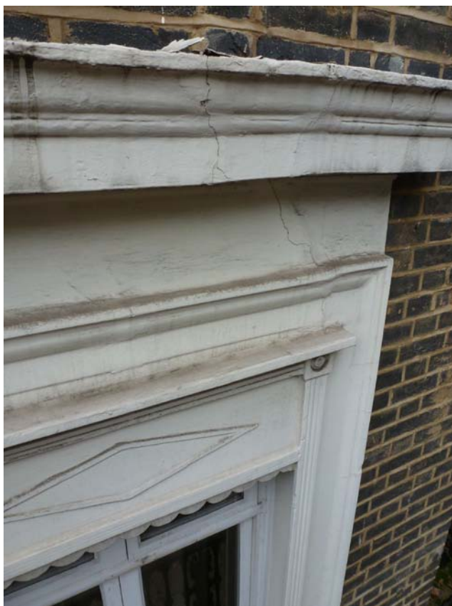
Photo 27: Taviton Annex - Regency balcony window blind box.
