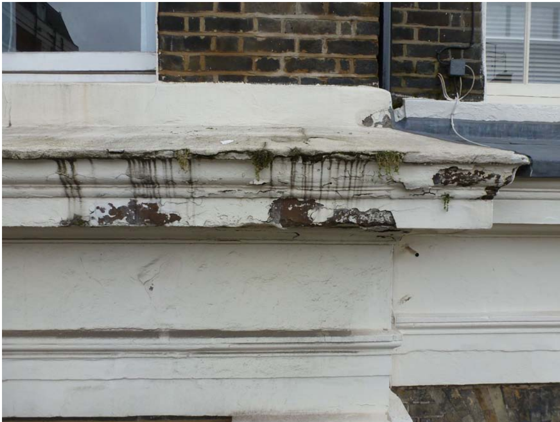
Photo 11: Endsleigh Street - main cornice band.
