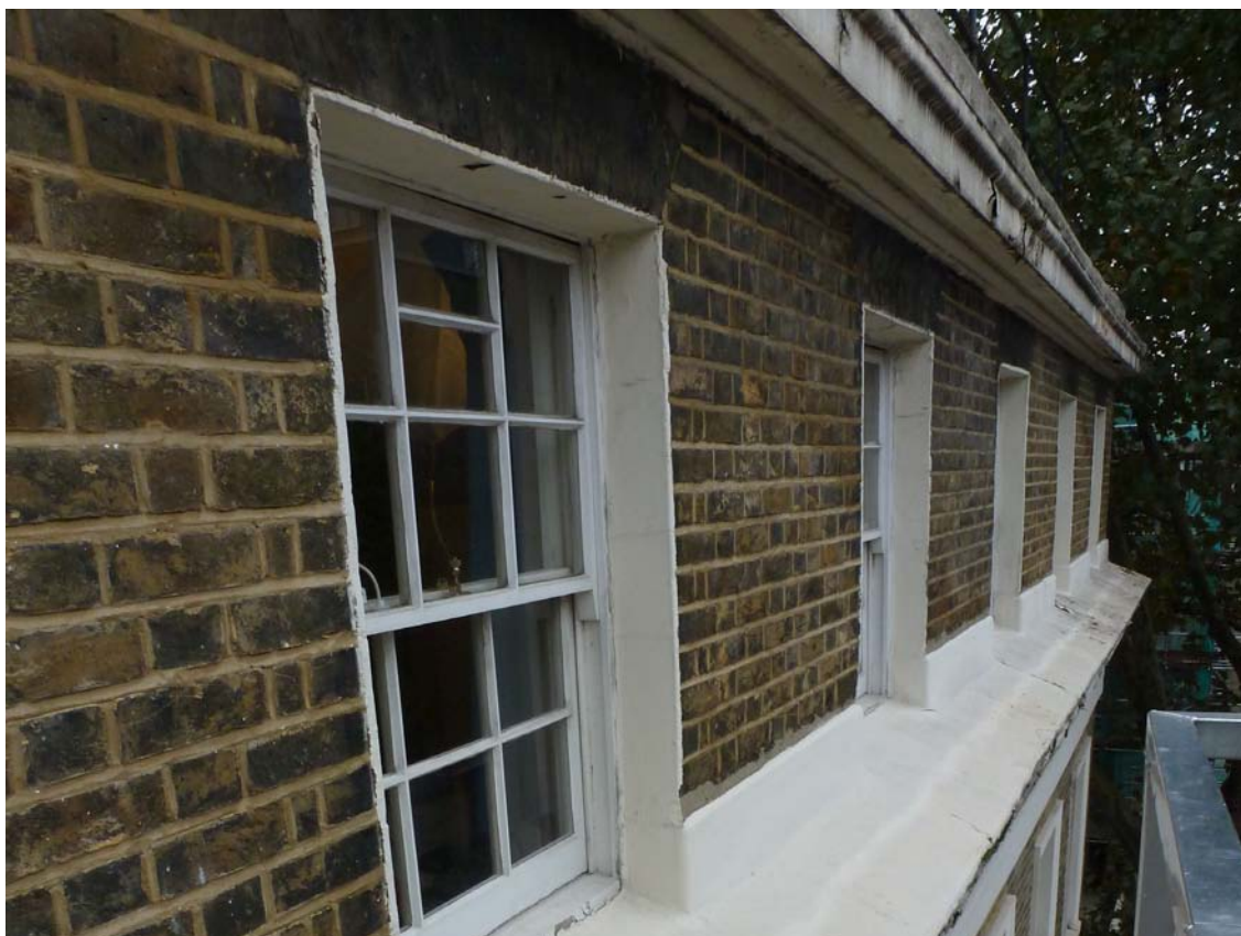
Photo 24: Taviton Annex - 3rd floor sash windows.
