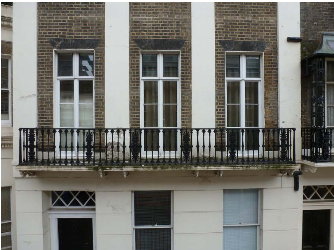
Photo 2: Endsleigh Street elevation.
