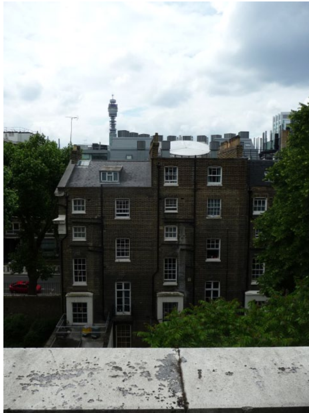
Photo 17: Taviton Annex: rear elevation
