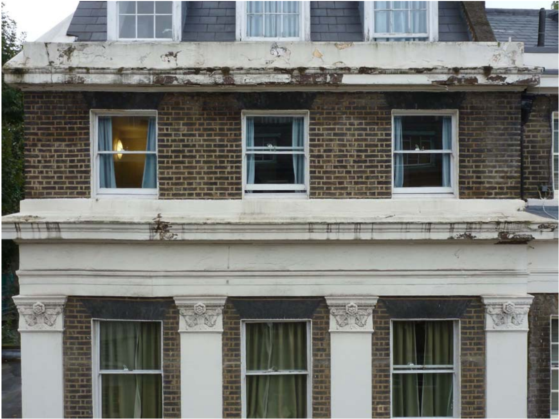
Photo 1: Endsleigh Street elevation.
