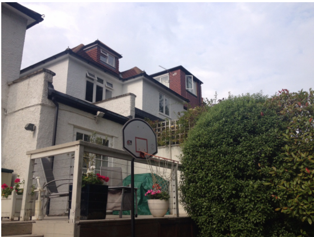
View towards number 72 Hillway, north of the application site
