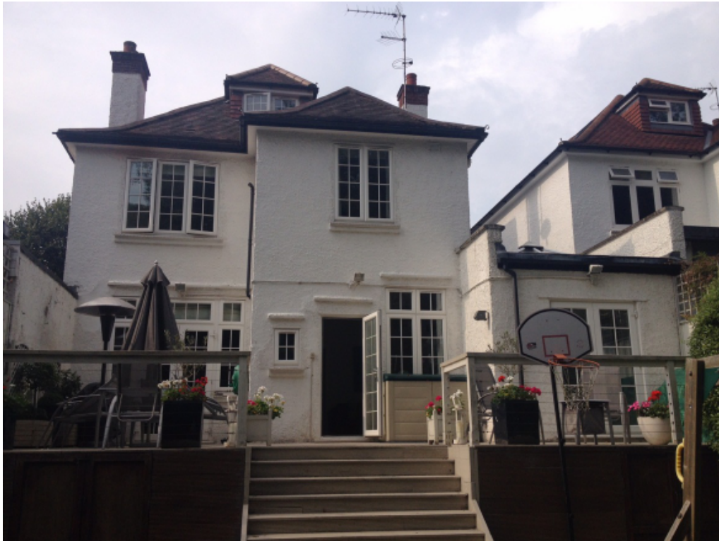
Rear elevation of application property
