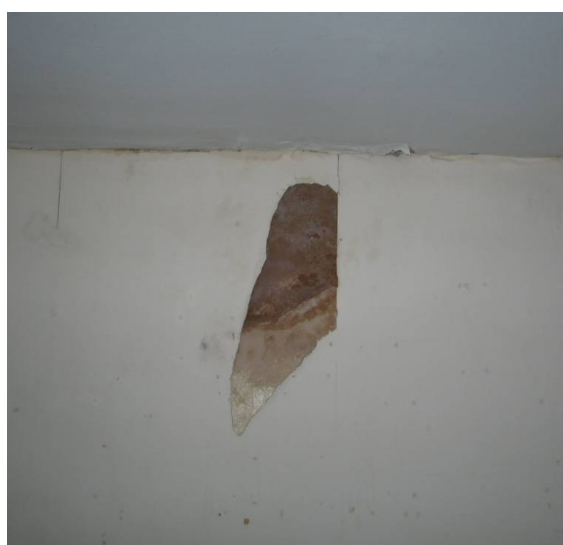
Bedroom F03, modern plaster repair (east external wall)
