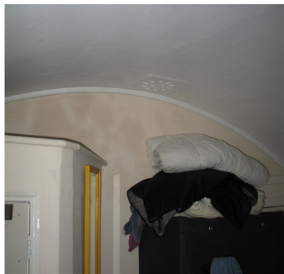
Bedroom F02, lobby partitions to be removed (fireboard on original door to be removed, and door reused)
