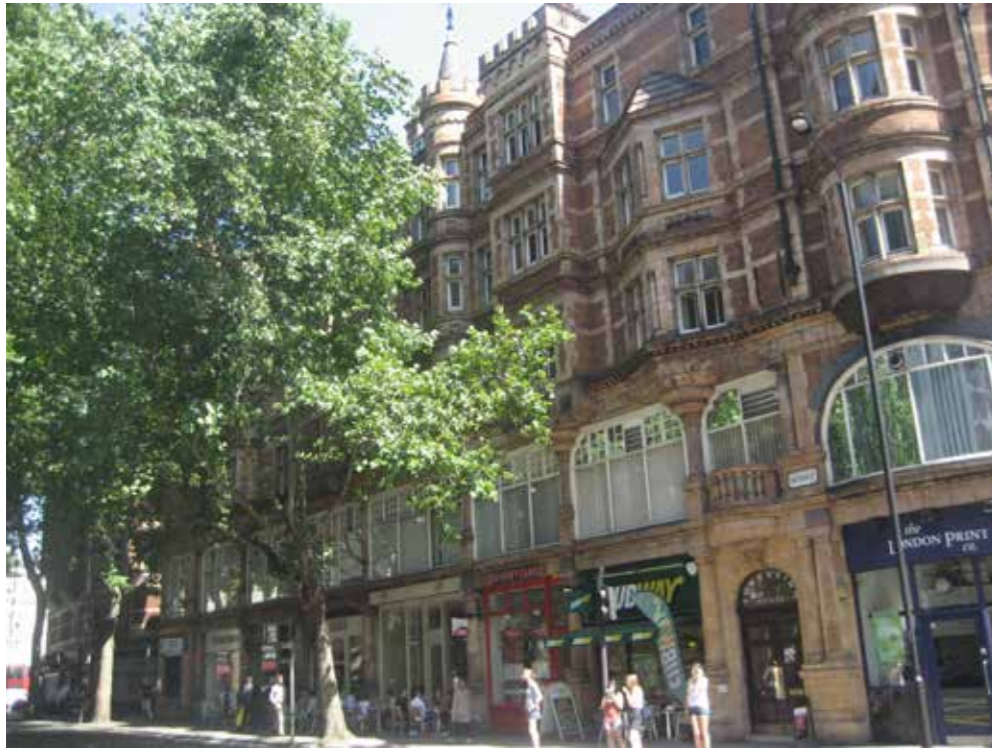
Fig. 6.6: Sovereign House frontage onto Shaftesbury Avenue.
