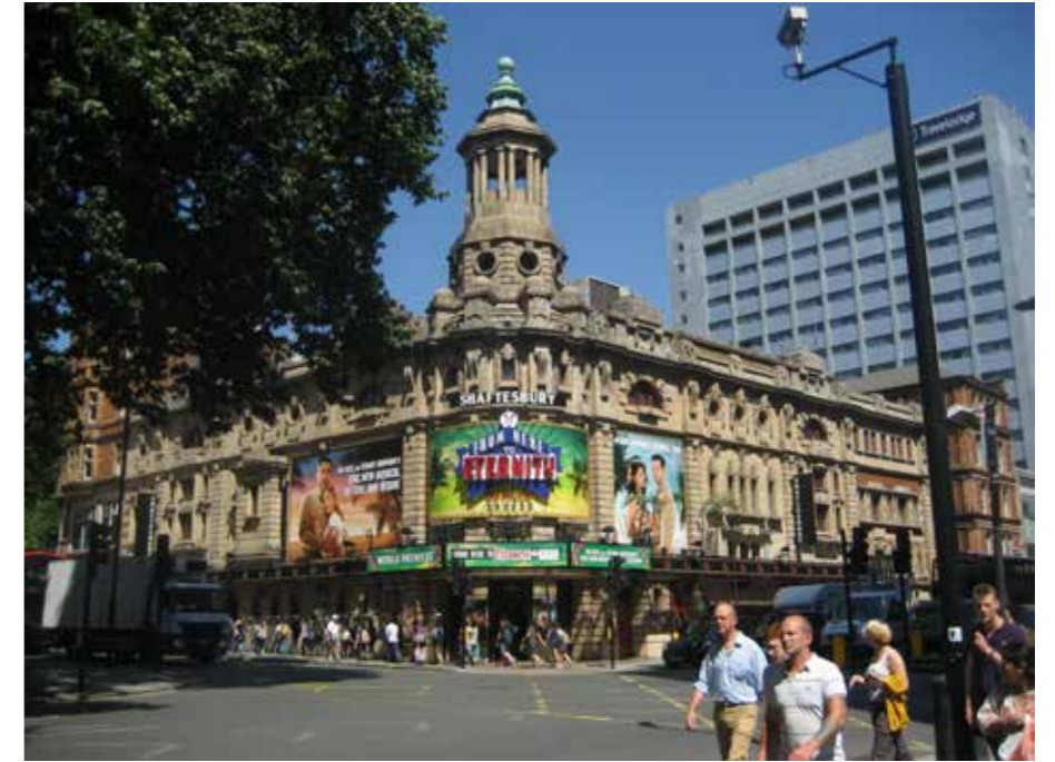
Fig. 4.11: Grade II listed Shaftesbury Theatre seen from the junction of Bloomsbury Street and St Giles High Street.
