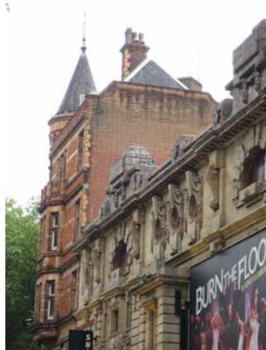
Fig. 4.10: Roofscape of Sovereign House and Shaftesbury Theatre.
