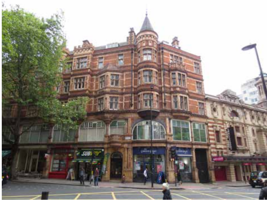
Fig. 4.9: Sovereign House seen from the junction of Shaftesbury Avenue and Bloomsbury Street. This is adjoined by Shaftesbury Theatre seen to its right.
