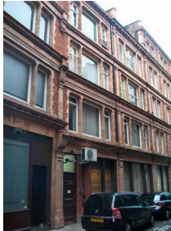
Fig. 8.3: (No. 2) 15 & 17 Grape Street, the Columbian Embassy adjacent to the subject site.
