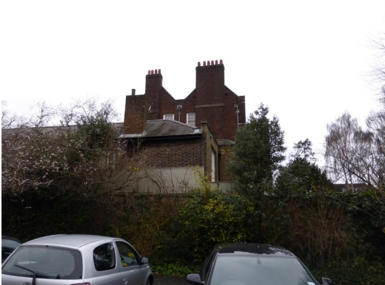
Figure 21: View towards site from car park of St Michael's Church
