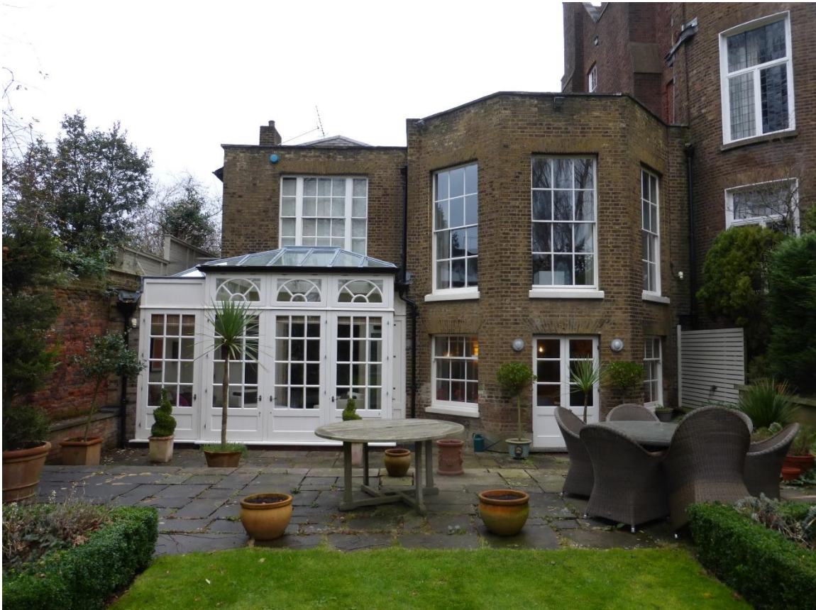
Figure 17: View of rear elevation
