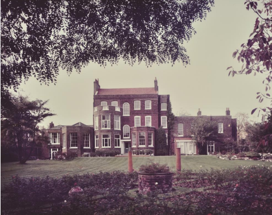
Figure 14: Rear elevation of Number Old Hall, 1983
