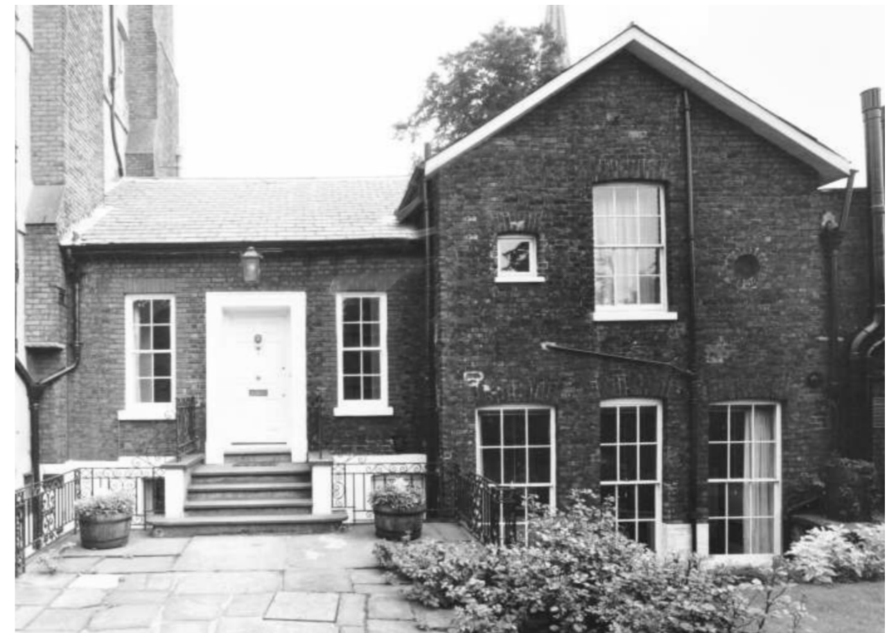
No. 1 Old Hall front facade in 1971, prior to the front extension construction
