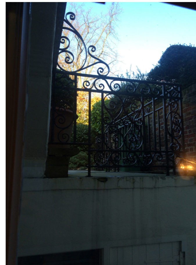
No. 1 lightwell railings
