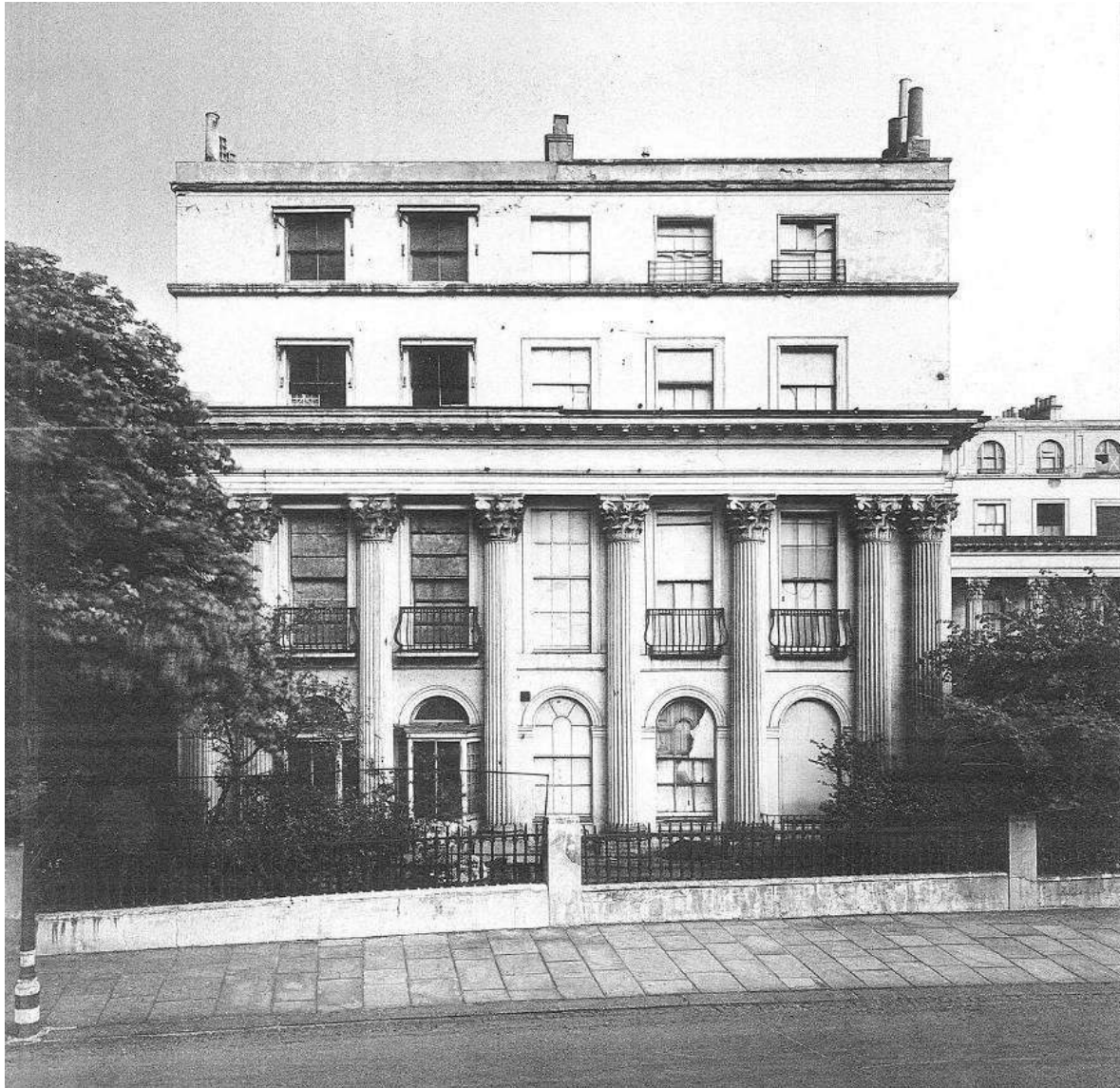
Figure 13: Photograph taken in 1943, shows 41 and 42, Regents Park elevation damage to the windows
