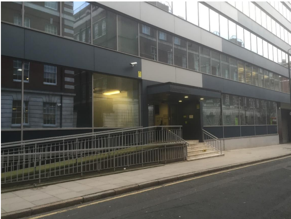
3. Main Entrance – Bidborough Street (Viewed from West)
