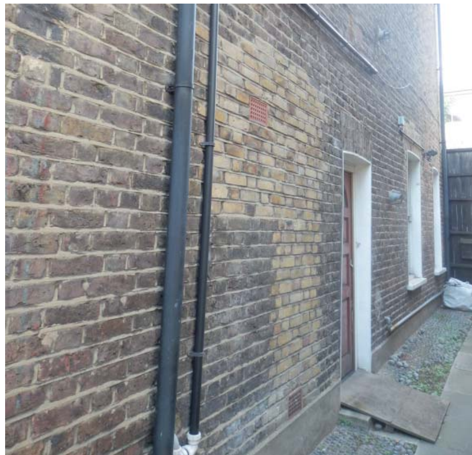
4. Access to apartment entrance
