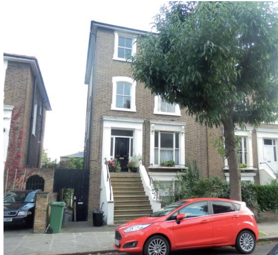
2. Front facade showing access to timber screen
