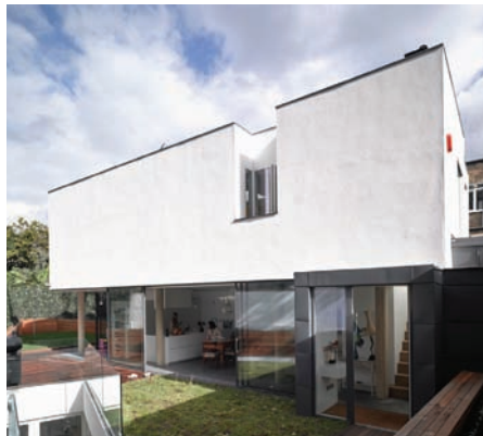
Work Sample 4: New Build in Camden Grafton Crescent, London,
