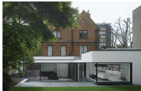
Work Sample 2: Contemporary extension to 7 Melbury House, London, W14
