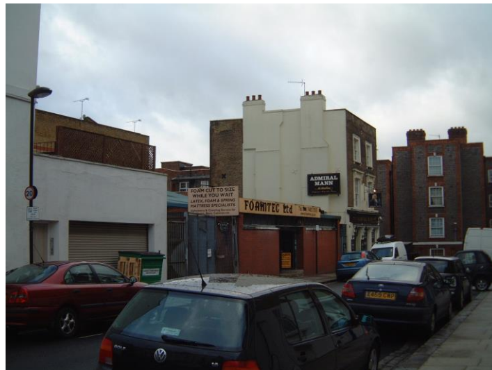
View towards Admiral Mann PH showing adjoining properties
