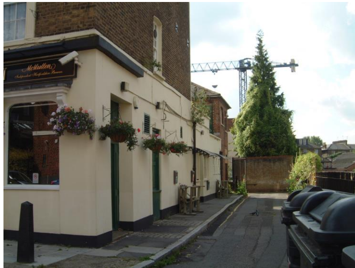
View along the side access road towards the rear of the property
