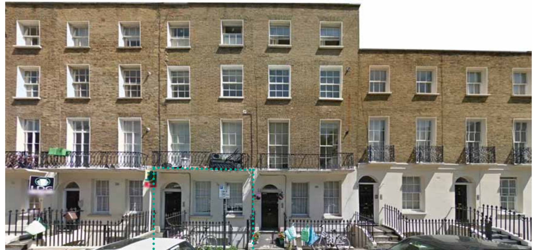
Front facades along Cloudesley Road
