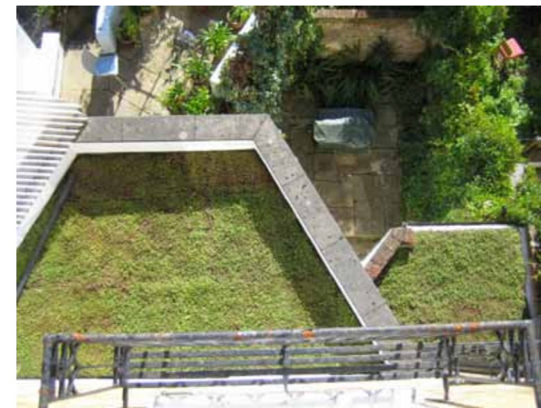
Low maintenance sedum roofs to rear extensions to a historic property.
