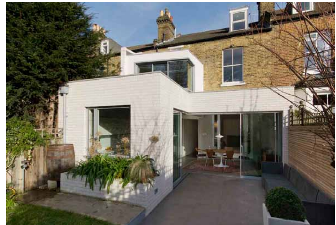
Example of a ground floor extension to a historic property in pale brick by Sam Tisdall Architects
