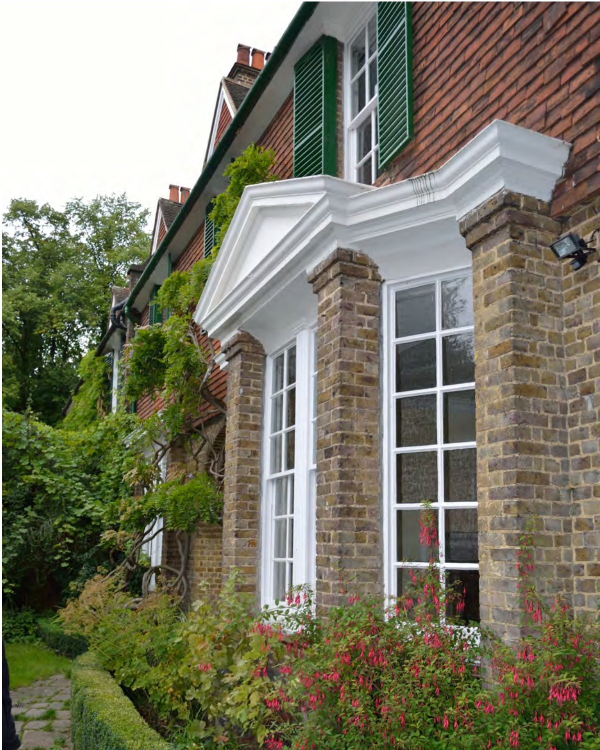
Fig 7. The drawing room bay window with its heavy pediment. Although well detailed, this bay window is an early 20th century addition probably replacing an identical window to that in the dining room.
