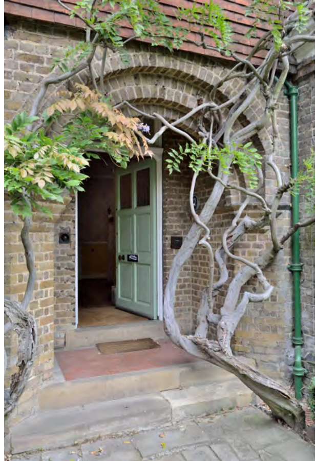
Fig 5, The front door showing the arched brick open porch—a typical Webb detail. The ancient wisteria may well be contemporary with the house.
