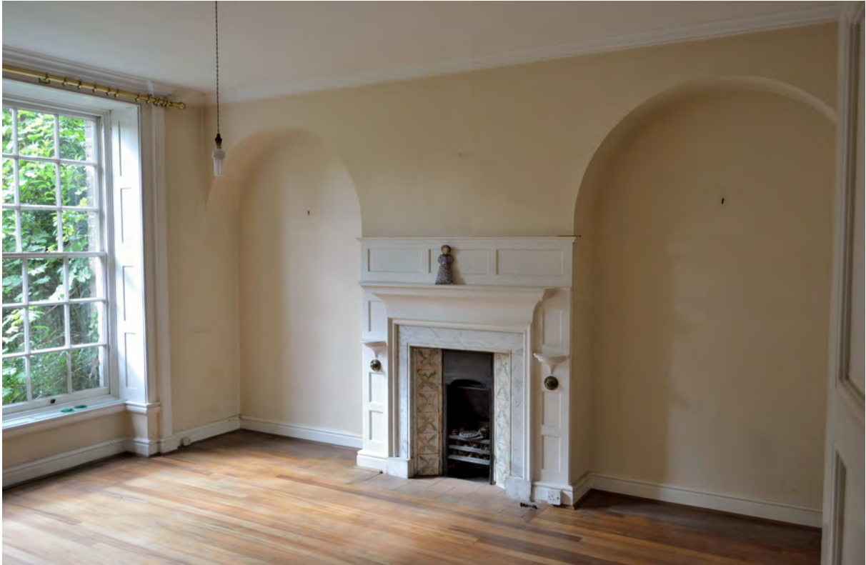
Fig 20. The dining room fireplace with adjacent alcoves which would have held matching furniture. On the opposite wall a larger alcove held a buffet. The floor is over-boarded with modern narrow boards, making the skirtings appear smaller than they really are.
