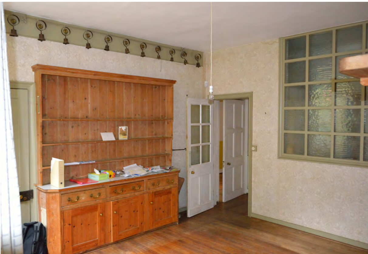
Fig 21. The kitchen dresser, which would originally have been painted, is believed to be original to the house. The modern over-boarded floor makes the skirtings appear mean, and the glazed partition forming the pantry is believed to be an early 20th century alteration.
