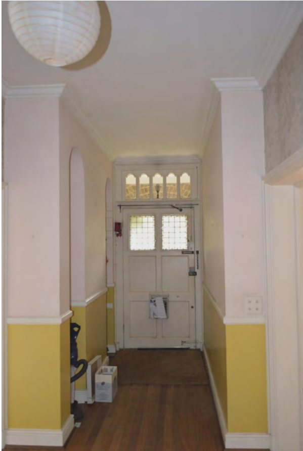
Fig 13, The entrance hall looking toward the front door. The floor is a modern over-boarded floor. Note the modern floorboards in the hall area.
