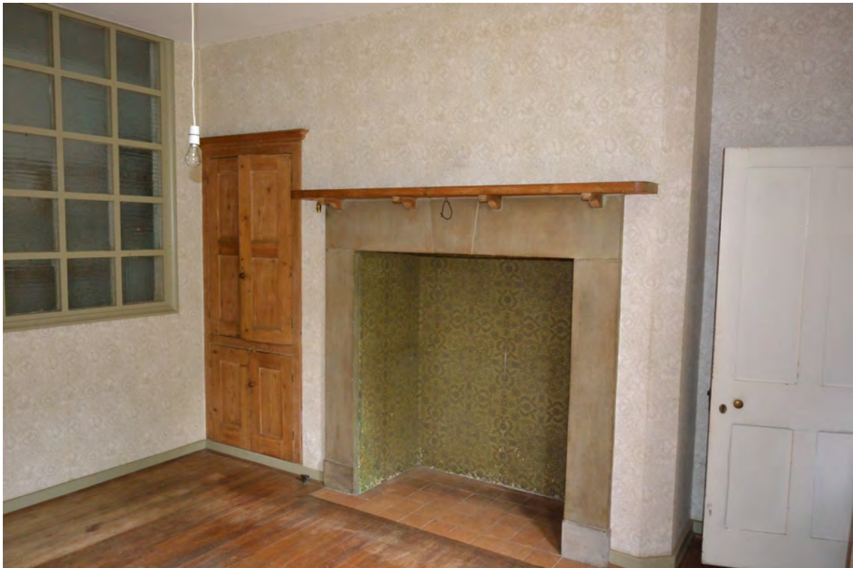
Fig 36, The kitchen fireplace with adjacent cupboard. Note how the screen to the pantry butts tightly up against it, the awkward relationship also suggests the partition may be a later insertion.
