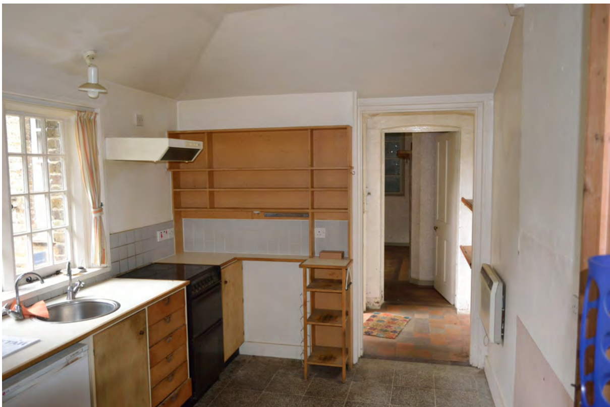
Fig 33, The converted scullery, now a kitchen. The walls have been dry-lined to reduce damp as the rear wall may be cut slightly into the hillside.
