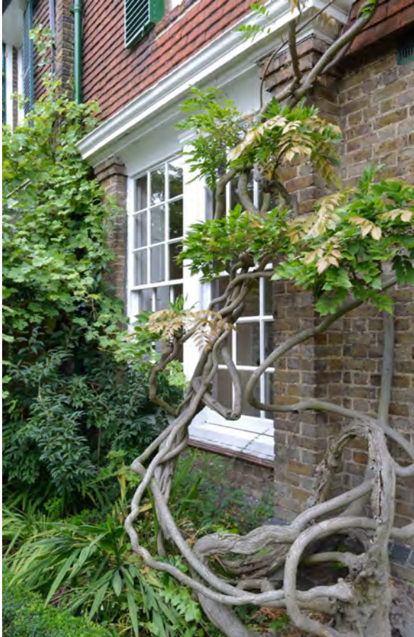
Fig 4, The slightly projecting dining room window has a pair of nine pane sashes beneath a deep cornice supported on brick pilasters.
