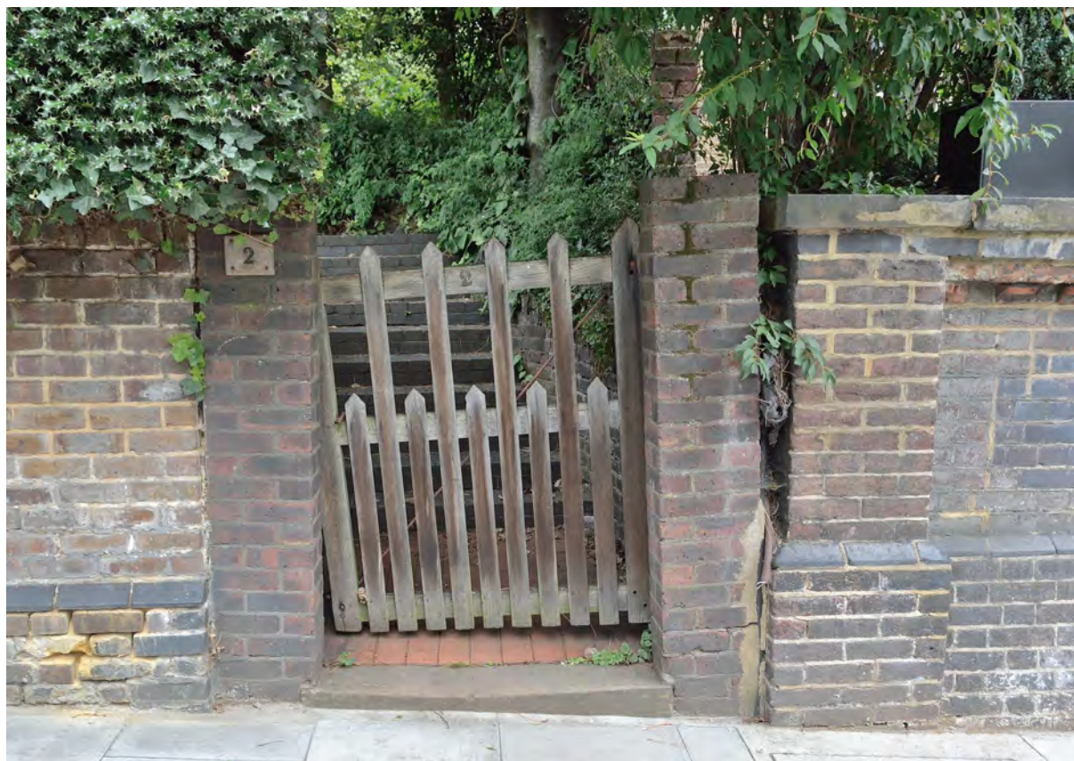
Fig 11. The simple wooden gate with the steps into the garden just visible beyond. The gate has been rehung but may reflect the detailing of the original wooden picket fence along the frontage, which was replaced by a brick wall in the early 20th century.
