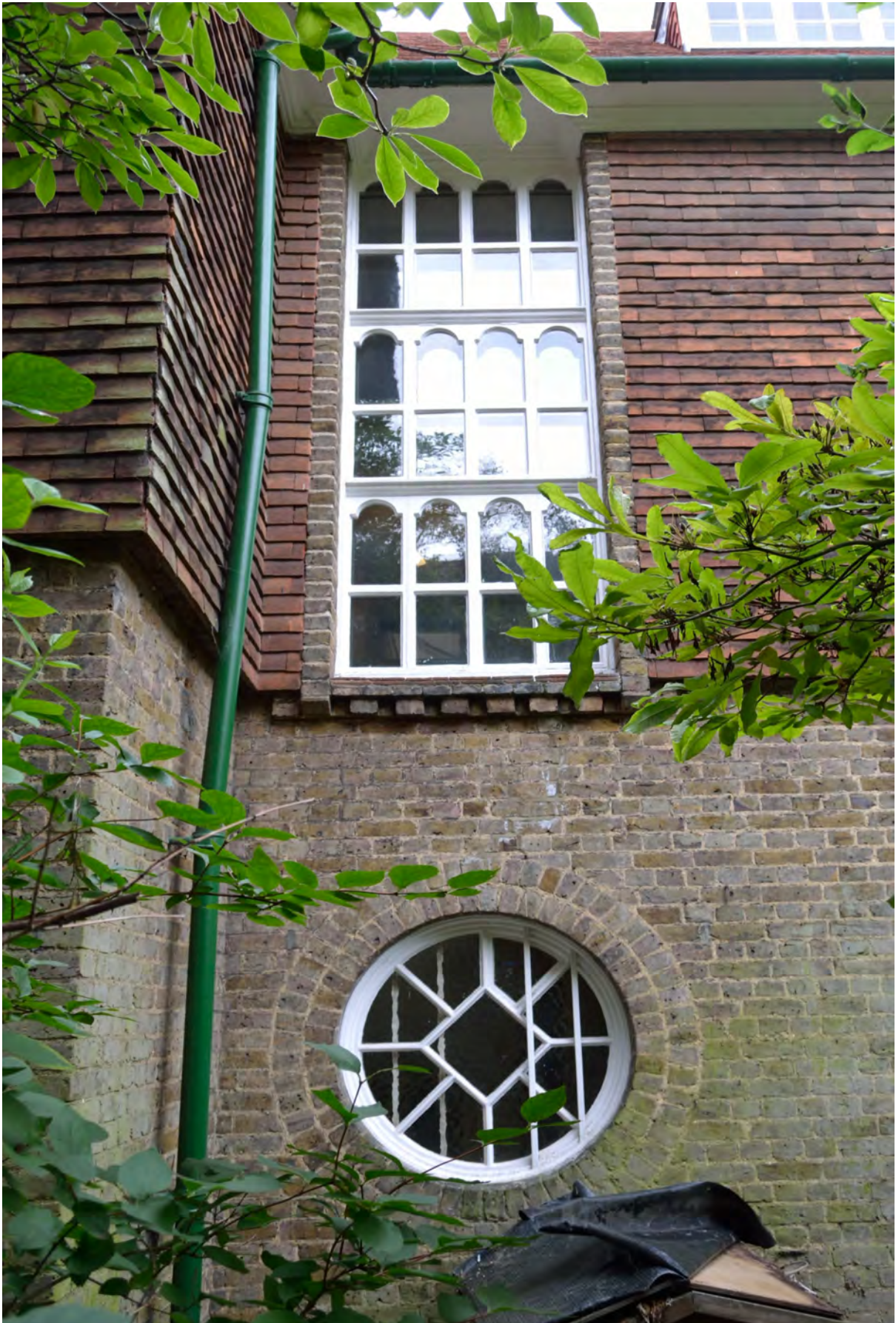
Fig 8. The .side elevation. Showing the narrower rear range containing the tall stair window above a round window lighting the WC, both typical Webb details. The wider front range contains the larger principal rooms
