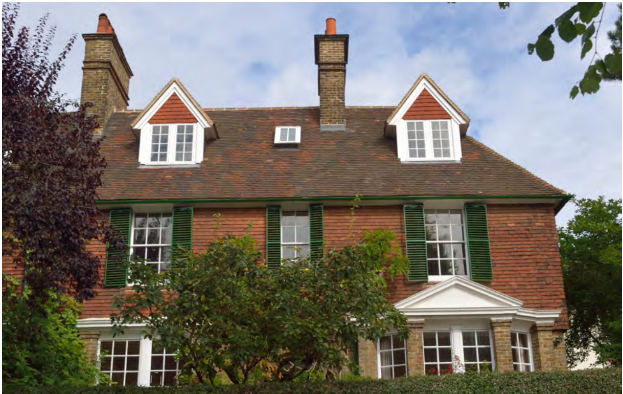
Fig 2, Detail of No 2 showing the (original) slightly projecting pair of nine pane sashes to the left (dining room) window and the later pedimented canted bay window with six pane sashes to the right (drawing room) .
