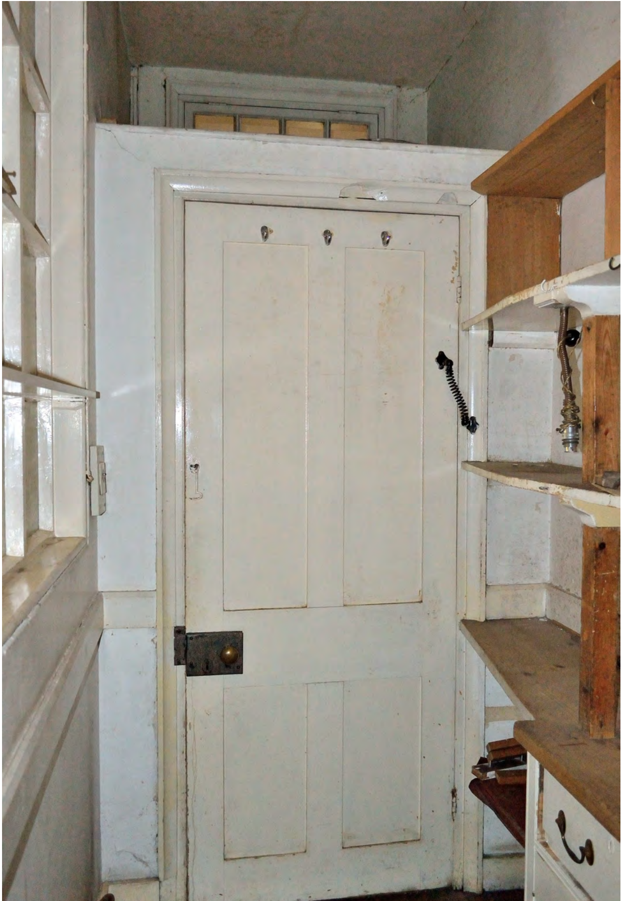
Fig 34, The pantry entrance lobby showing its awkward form. The window to the left appears to be a modern insertion , originally it only had borrowed light from over the kitchen door seen above the lobby.
