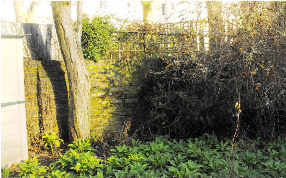
Figure 3: Third pier and adjacent tree.
