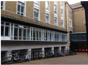
Physics Building Elevation facing rear services yard
