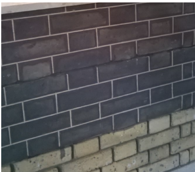
Site Sample 1 - Tuck pointing / brick staining
