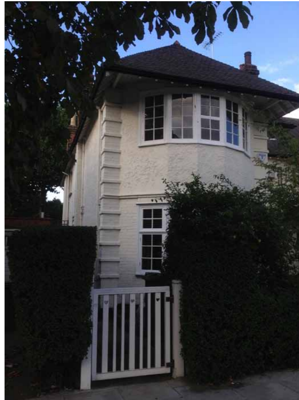
View looking North showing Front Facade
