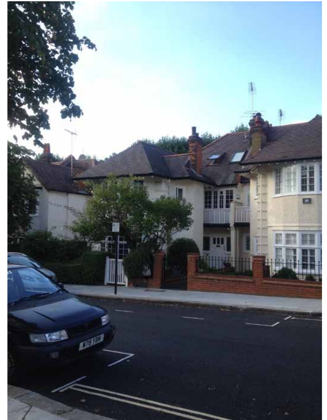
View looking West showing Front Facade
