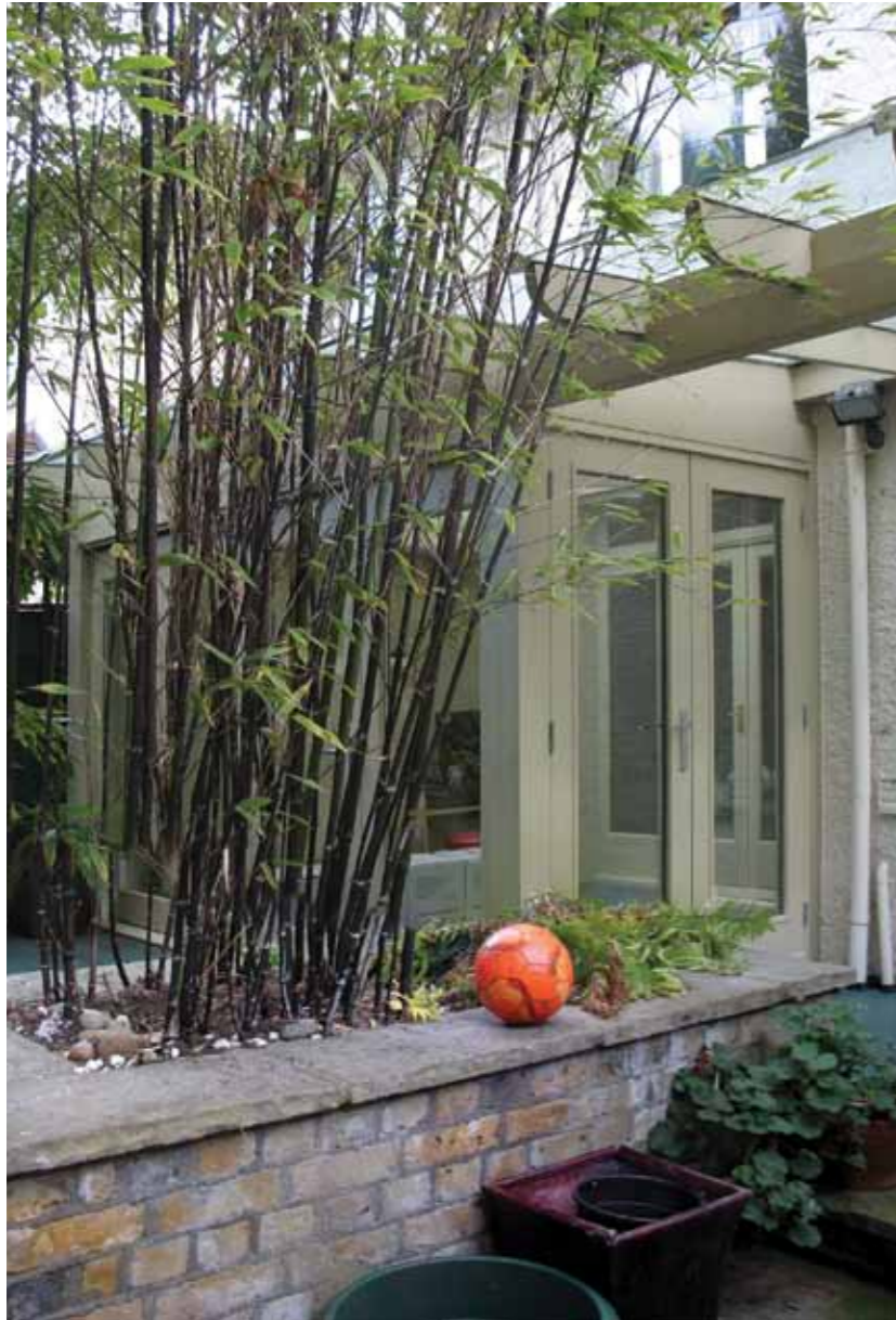
View looking East showing existing Rear Extension
