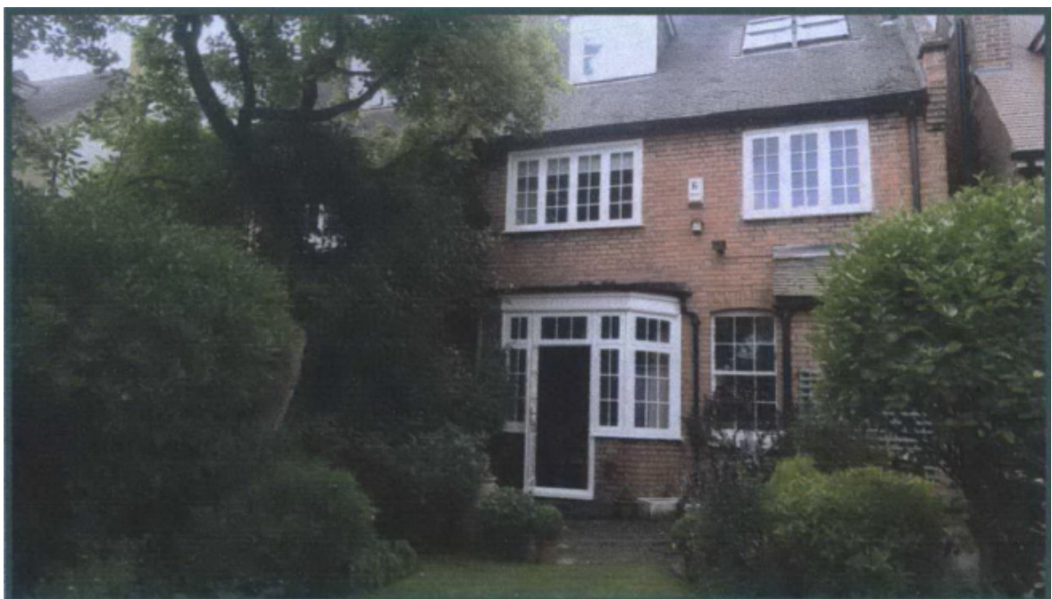
Photograph 4: Existing canopy encroachment from T1 (Source: ATS Report)
