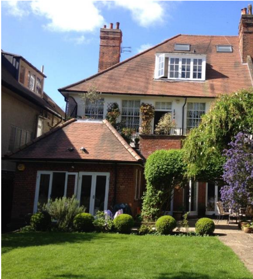
View of the rear of No. 3
