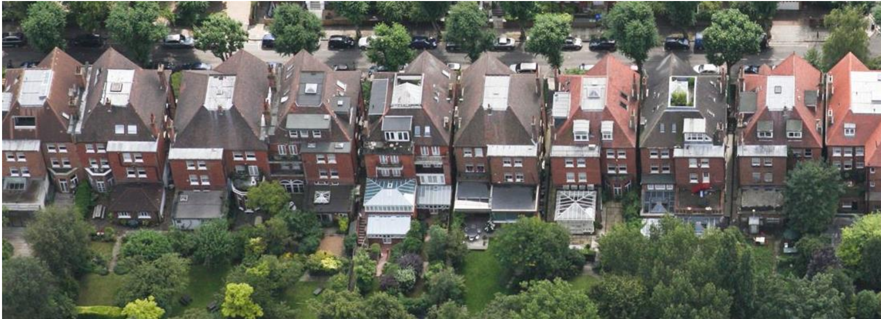
View along Wedderburn Road which runs parallel to Akenside Road
