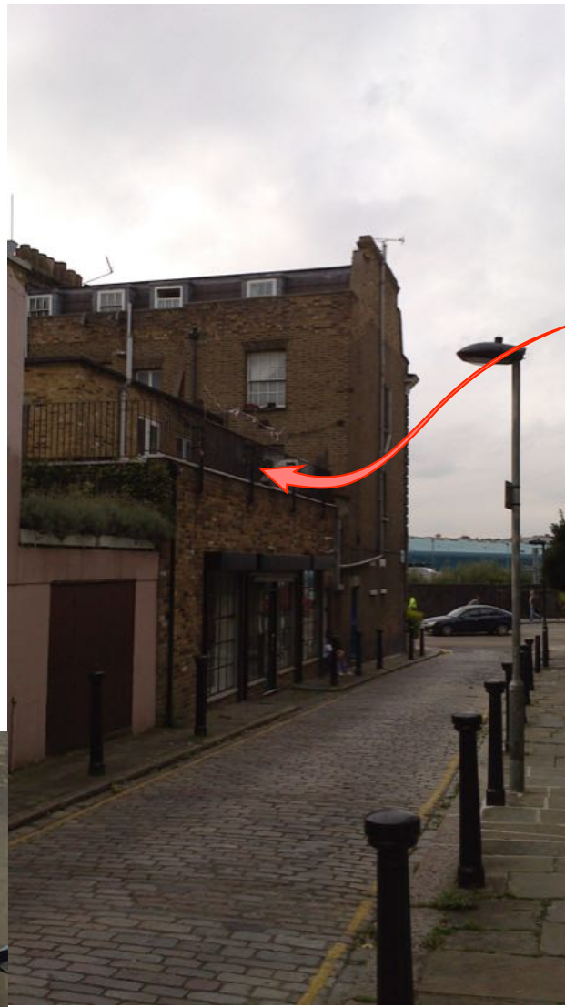
View of rear tenement site on Leverton Place showing the set back first floor accommodation
