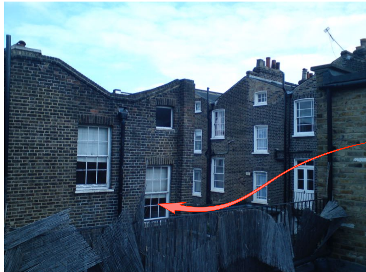
View at roof level of adjacent buildings to the south
