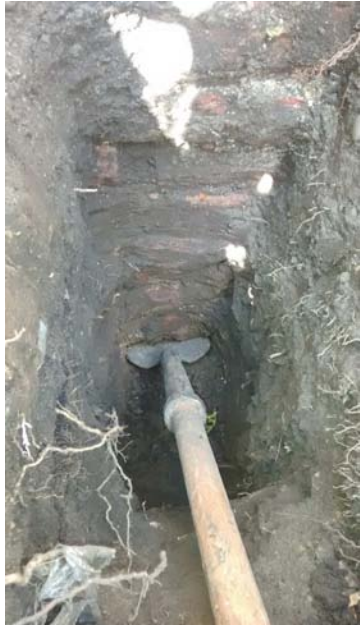
Photo showing TP2
