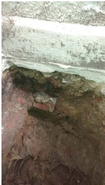
Brick foundation on right hand side of TP1.
