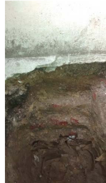
Brick Corbels on left hand section of TP1.
