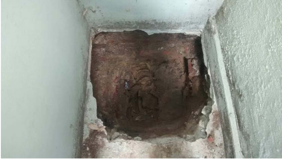
Photo showing TP1.
