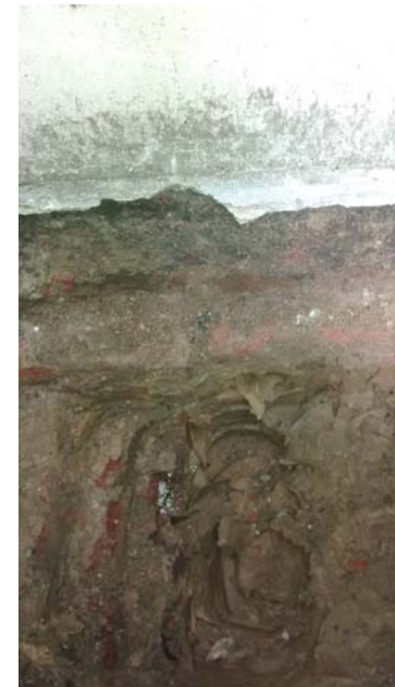
Brick foundation in central section of TP1.
