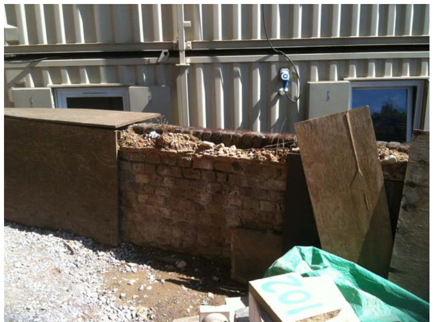
Photo 3: Looking South from the house side of the wall
