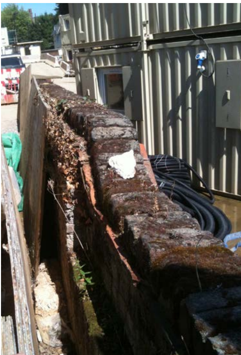
Photo 1: Looking along coping to the East.
